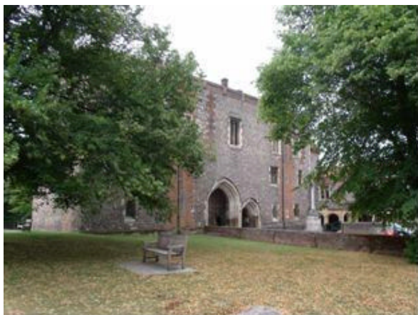
The Abbey Gateway is now part of the school. Percival Blow's 1920s school buildings link to the Gateway through the use of similar materials and Gothic architecture.
