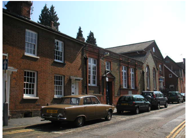
Local red brick is the most common material but yellow and purple (Luton grey) brick is also used.
