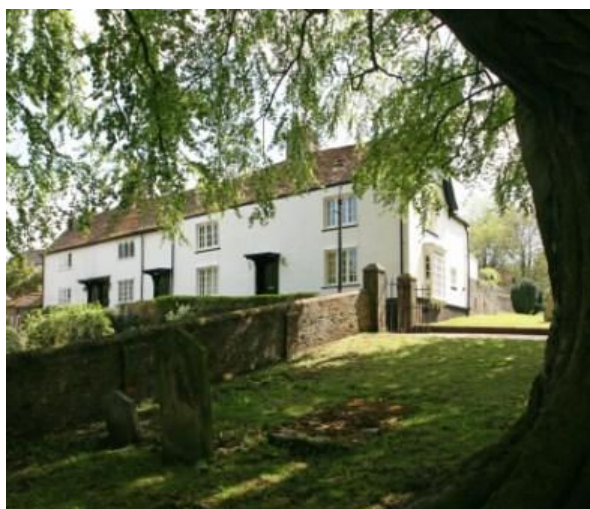
Romeland Cottages have a jettied timber frame and, typically for this area and the adjoining area 4c, they have been refaced at a later date. Image courtesy of John Bethel.
