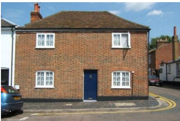
Most of the buildings in this character area are located on the pavement edge.
