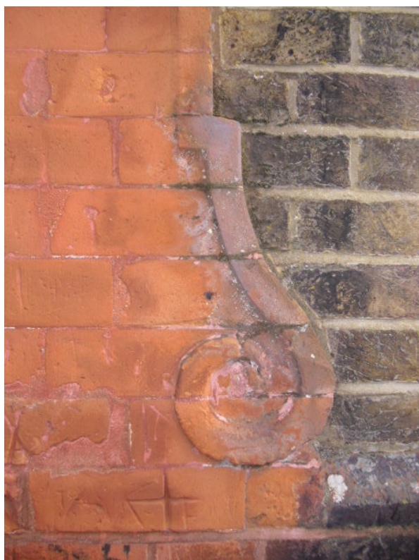
Many of the buildings exhibit interesting and high quality architectural detailing.
