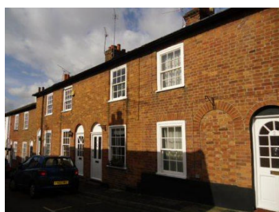
Small-scale cottages in Queen Street.
