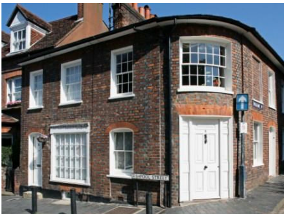
Most of the windows and doors are traditional timber and some buildings display interesting fenestration like this curved window to fit the curved corner. Image courtesy of John Bethell.
