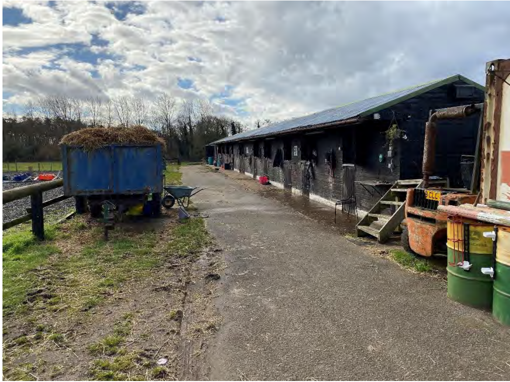
Plate 2: Stables within the Site, view to south-west
