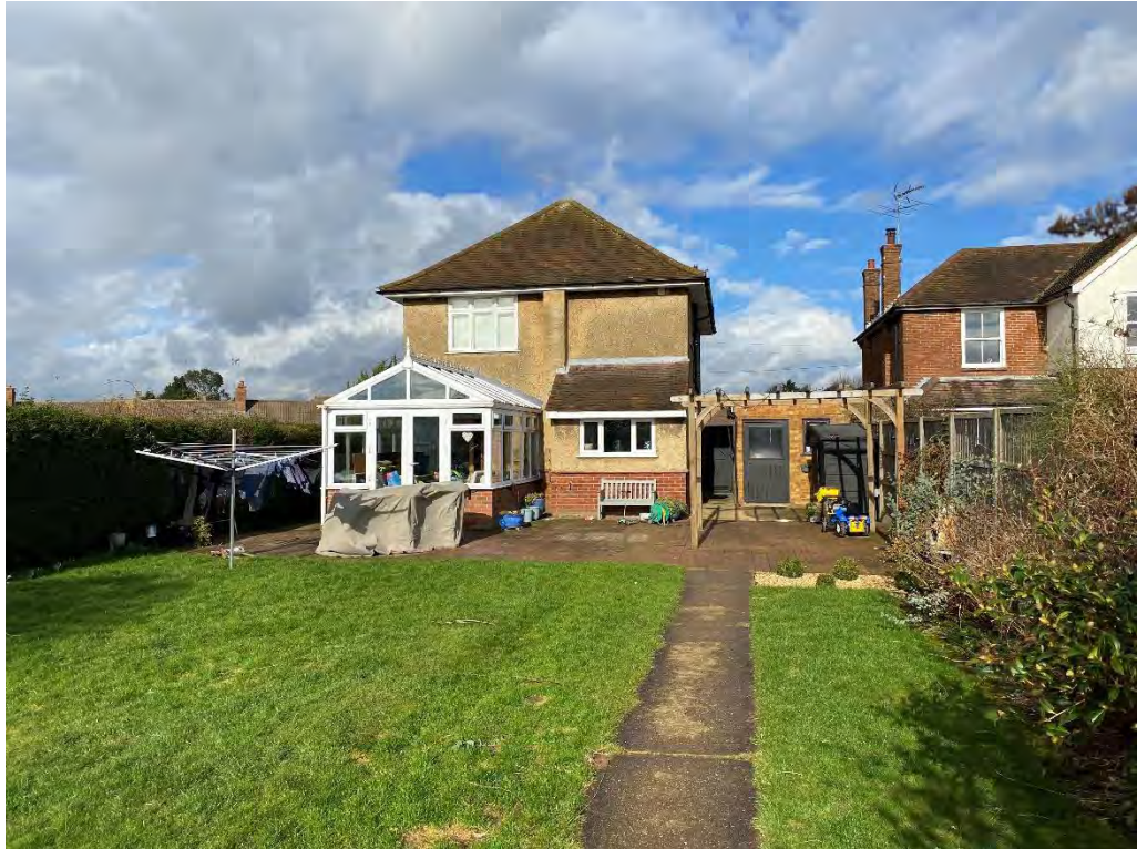
Plate 4: View of rear of No. 42 Tollgate Road, view to north
