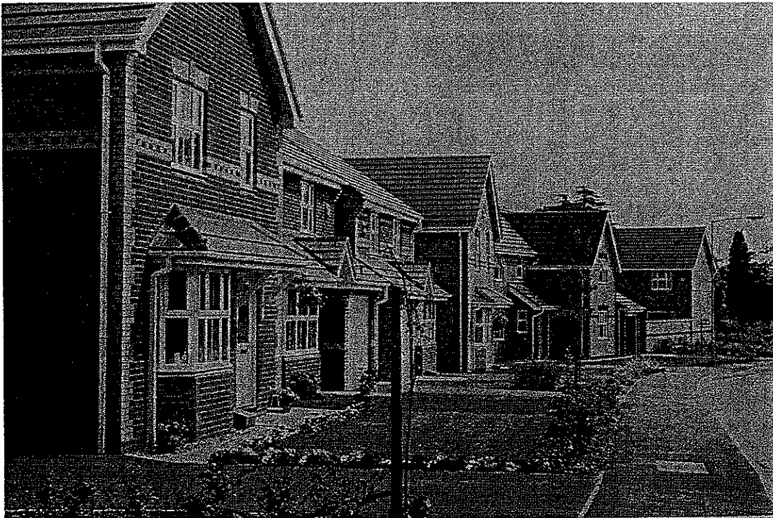
Figure 24 | New housing benefiting from defensible space
