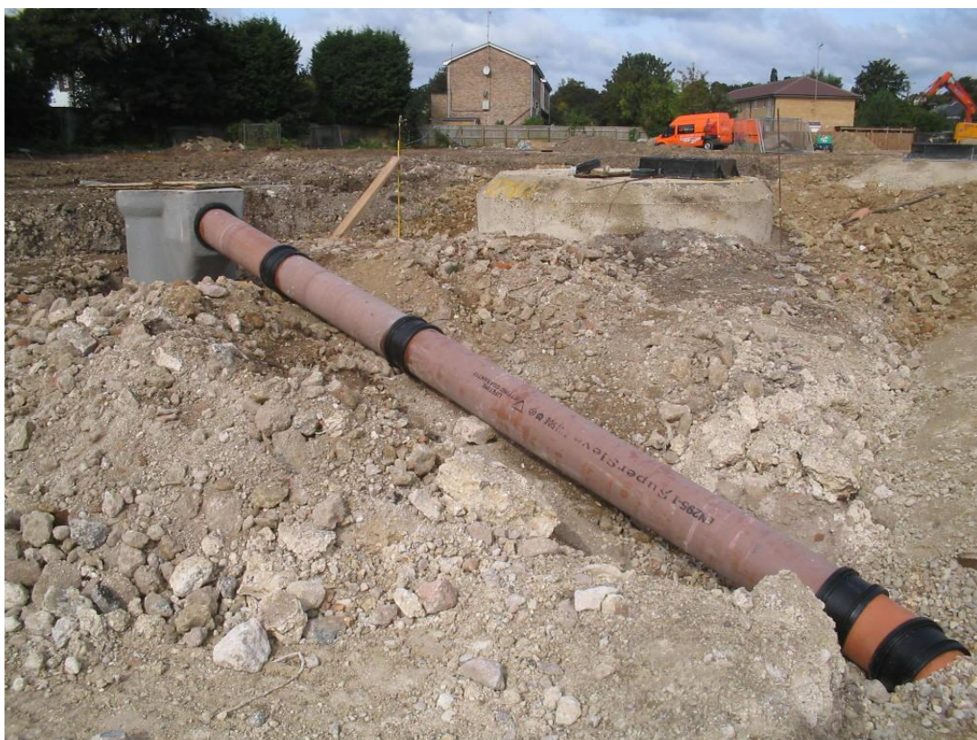
Photo 4.4.1.1: Gully Construction
