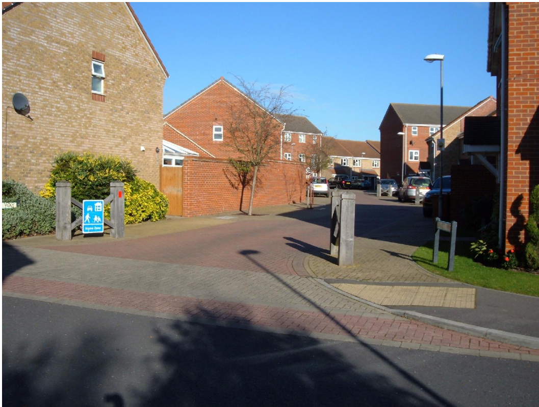
Photo 4.1.3.1: Entrance to a 20mph zone with raised 'gateway' feature
