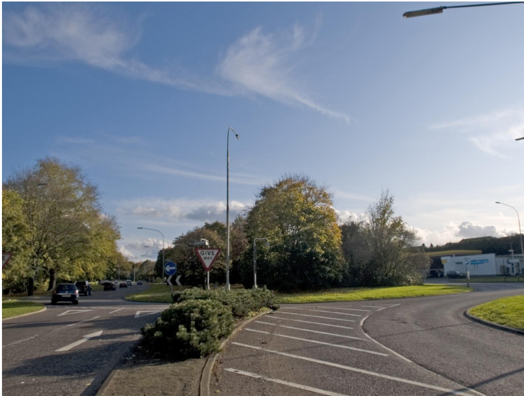
Photo 4.2.1.1: Example of a normal roundabout
