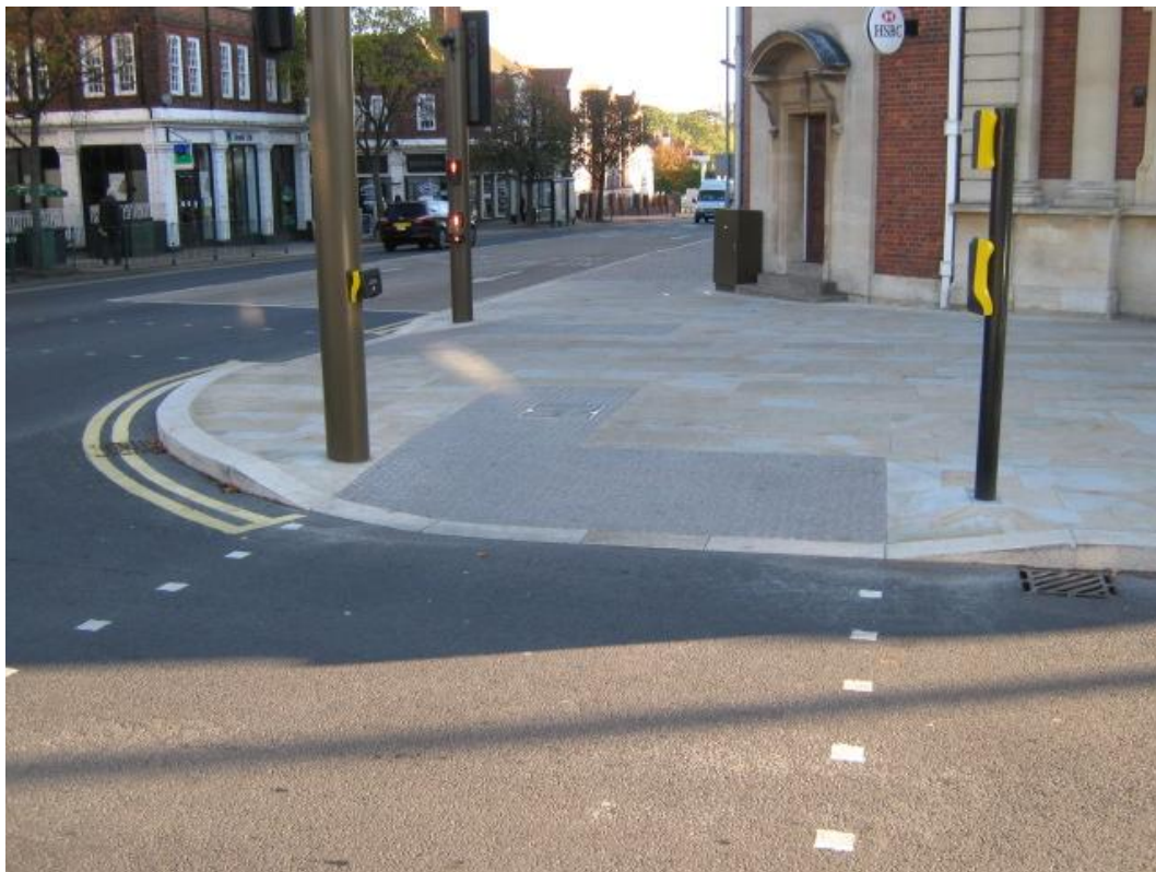
Photo 4.11.3.1: A controlled pedestrian crossing
