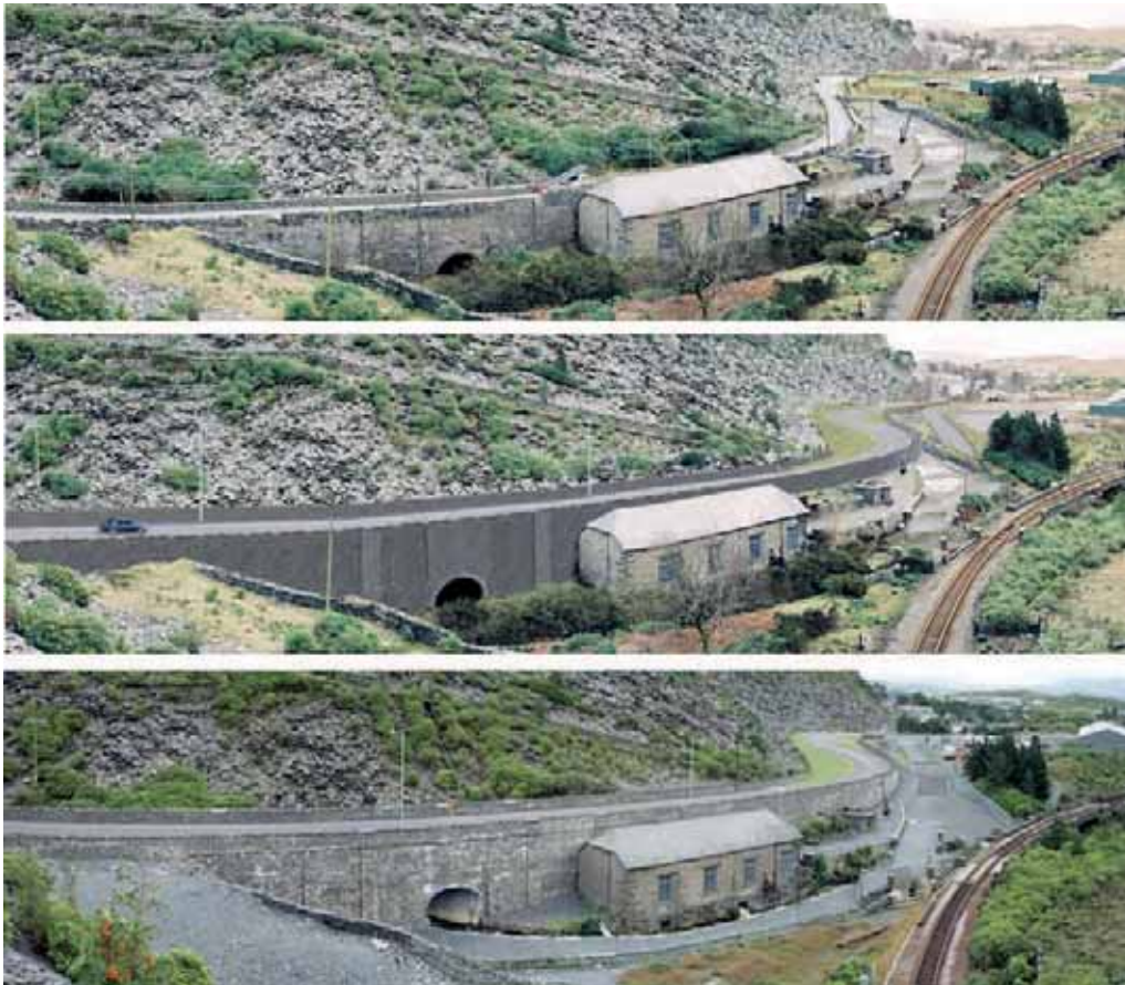
Figure 8.5 Review and monitoring: what actually happened compared with what was predicted in the LVIA
