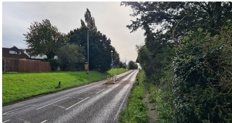
Figure 2-2 - View of the narrow footway to the south of the proposed access
