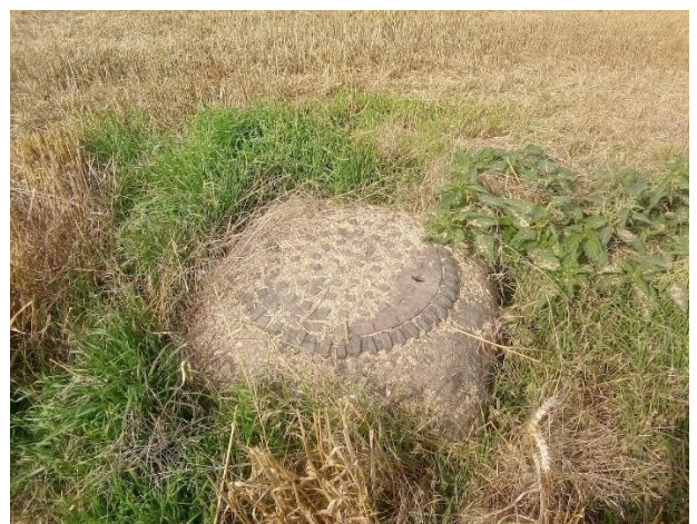
Figure 2.6: Manhole and inspection pit for sewer line running across the site.
