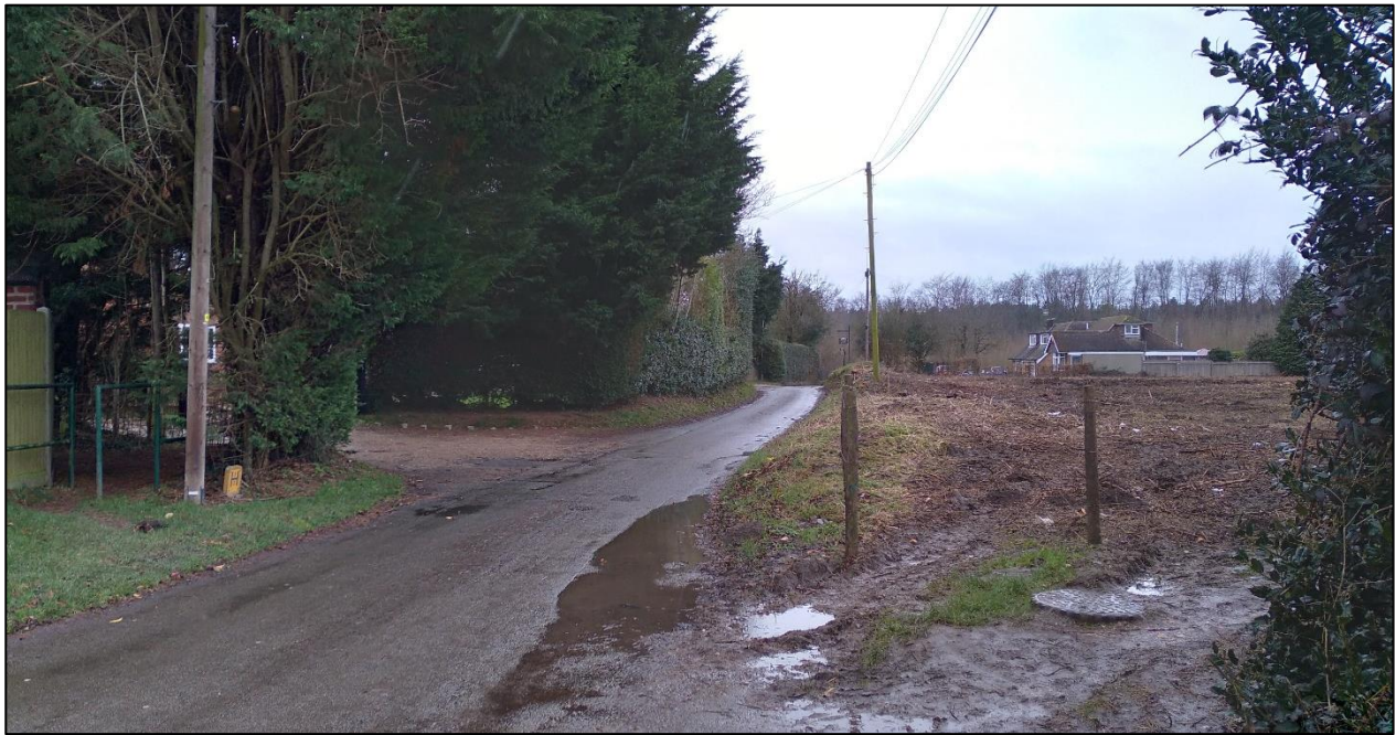
Figure 10: Ragged Hall Lane (looking west)
