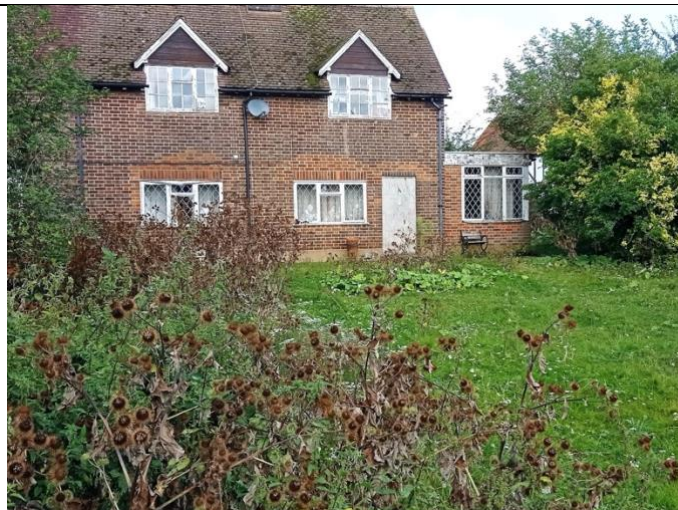
Photograph 1: Southern elevation of B1 in the north-east of the site (Moderate bat potential)
