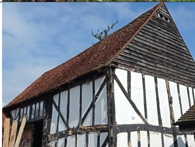
Photograph 2: South-western elevation of B5 in the north-east of the site (high bat potential)
