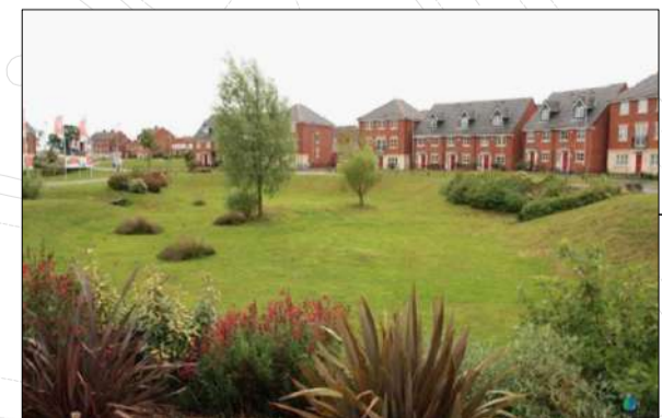
Infiltration / Attenuation Basin
