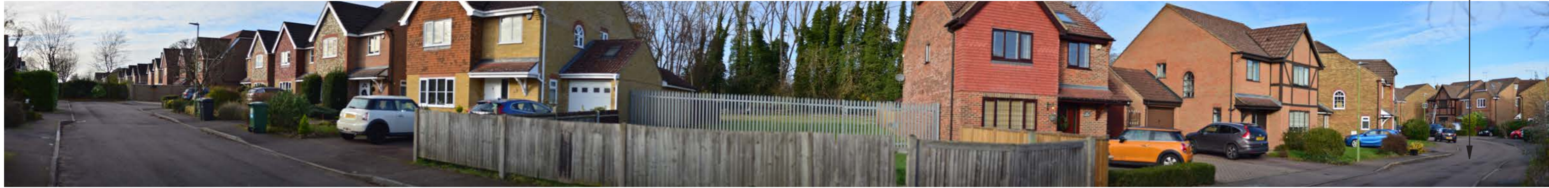
SITE CONTEXT PHOTOGRAPH 1: VIEW NORTH-WEST FROM BETWEEN 46 AND 50 FORGE END PANORAMIC PHOTOGRAPH: NOT TO SCALE AND FOR CONTEXT ONLY
