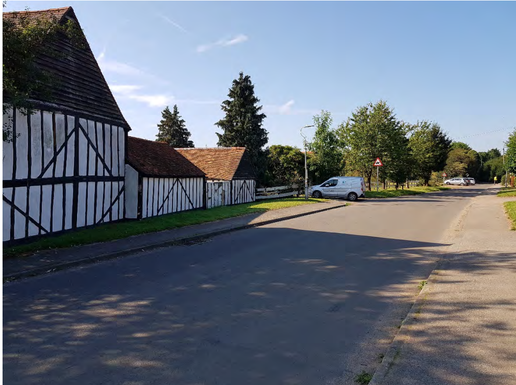
Plate 30: View of the farmyard section from Chiswell Green Road.
