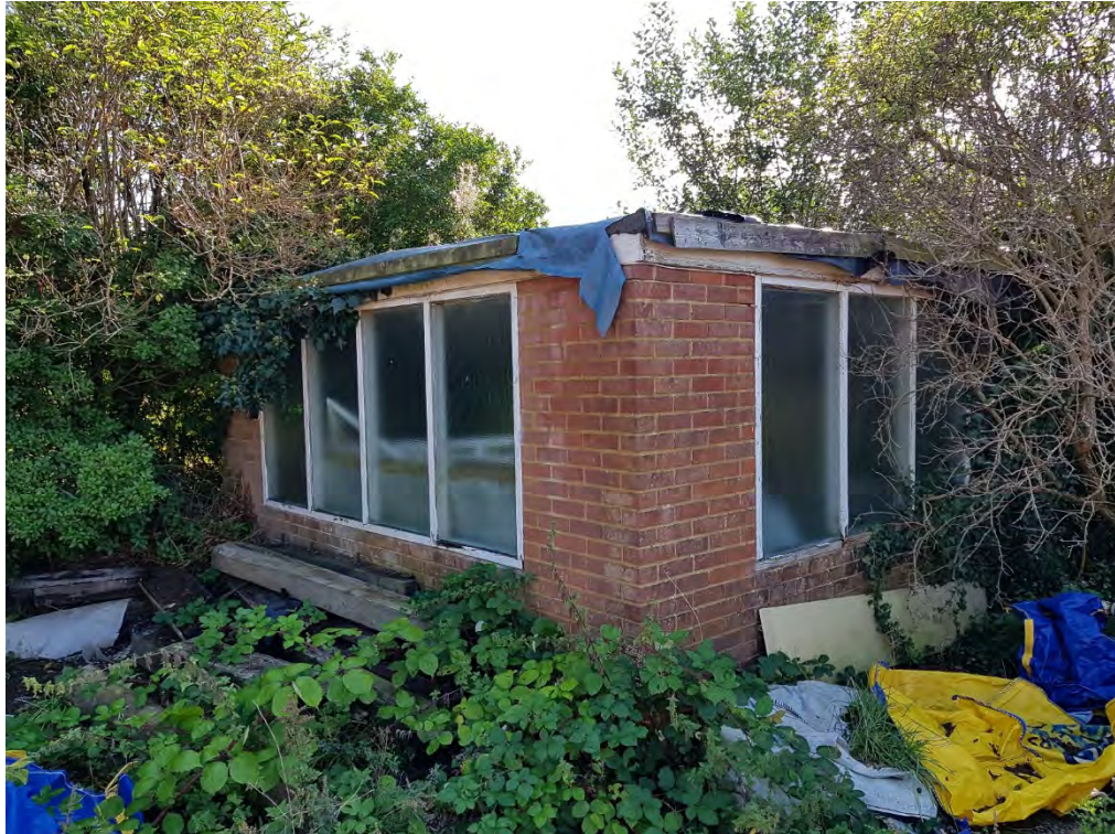
Plate 25: Possible boiler room or changing rooms for the former swimming pool.
