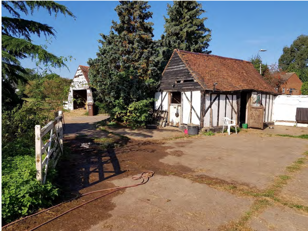
Plate 23: Timber framed sheds either side of the farm yard entrance.
