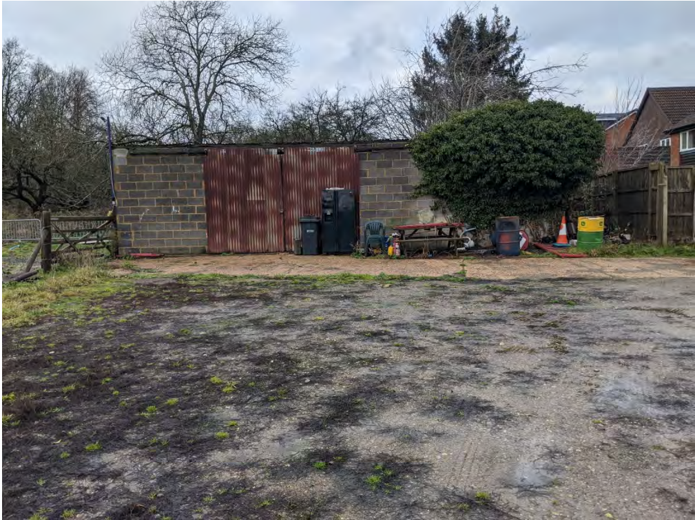
Plate 1: A breezeblock building with corrugated metal doors adjacent to the access way from Forge End on the eastern boundary.
