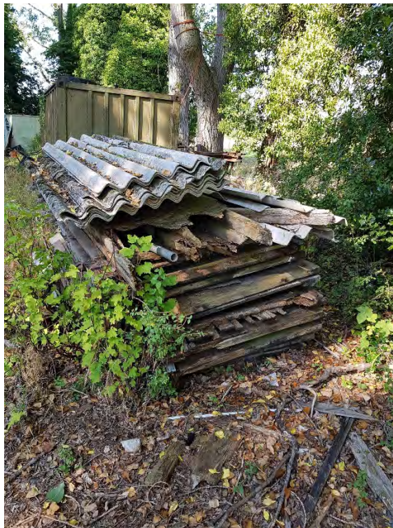
Plate 10: Stacked asbestos cement sheeting in the south eastern section of the site.
