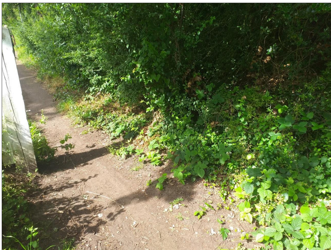
Photo 1 – western side of Park Street Lane by the “Welcome to Park Street” picket gates, looking southwards. Whilst, because of its overgrown nature, the drainage ditch is unclear from this photograph, on the ground its presence is obvious.
