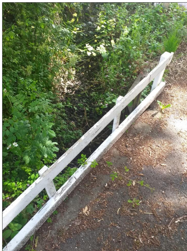
Photo 3 – culverting on western side of Park Street Lane
