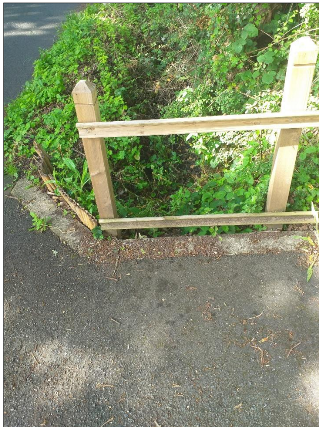
Photo 2 – culverting on western side of Park Street Lane
