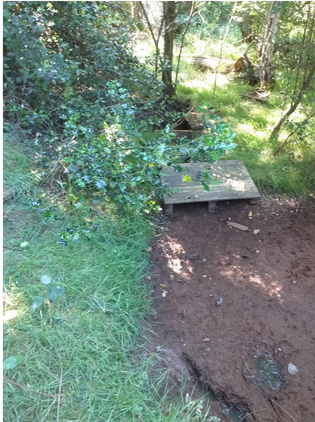
Photo 2: an area where water appears to have pooled in the past, identified by a blue circle on Ditch 2 (Appendix 1). The bed was very boggy and did not take my weight (hence the two footprints which subsequently filled with water). A concrete catchpit can be seen on the far side of the 'bridge'.
