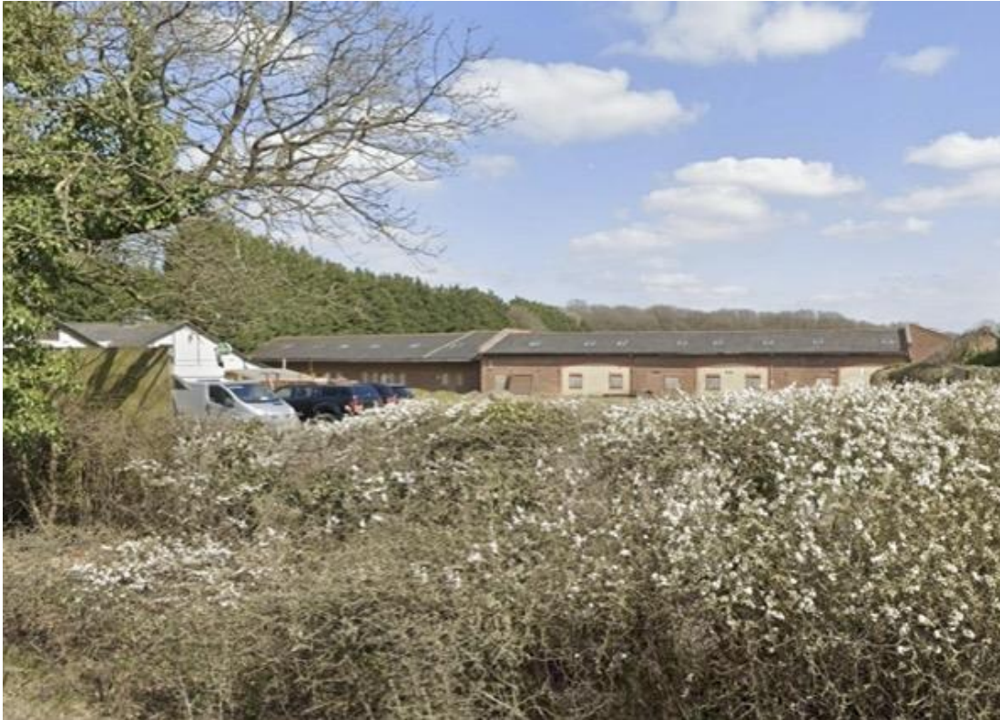
Building C and part of Building B viewed from Lye Lane
