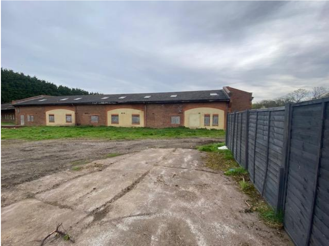
Building C viewed from the Site Frontage
