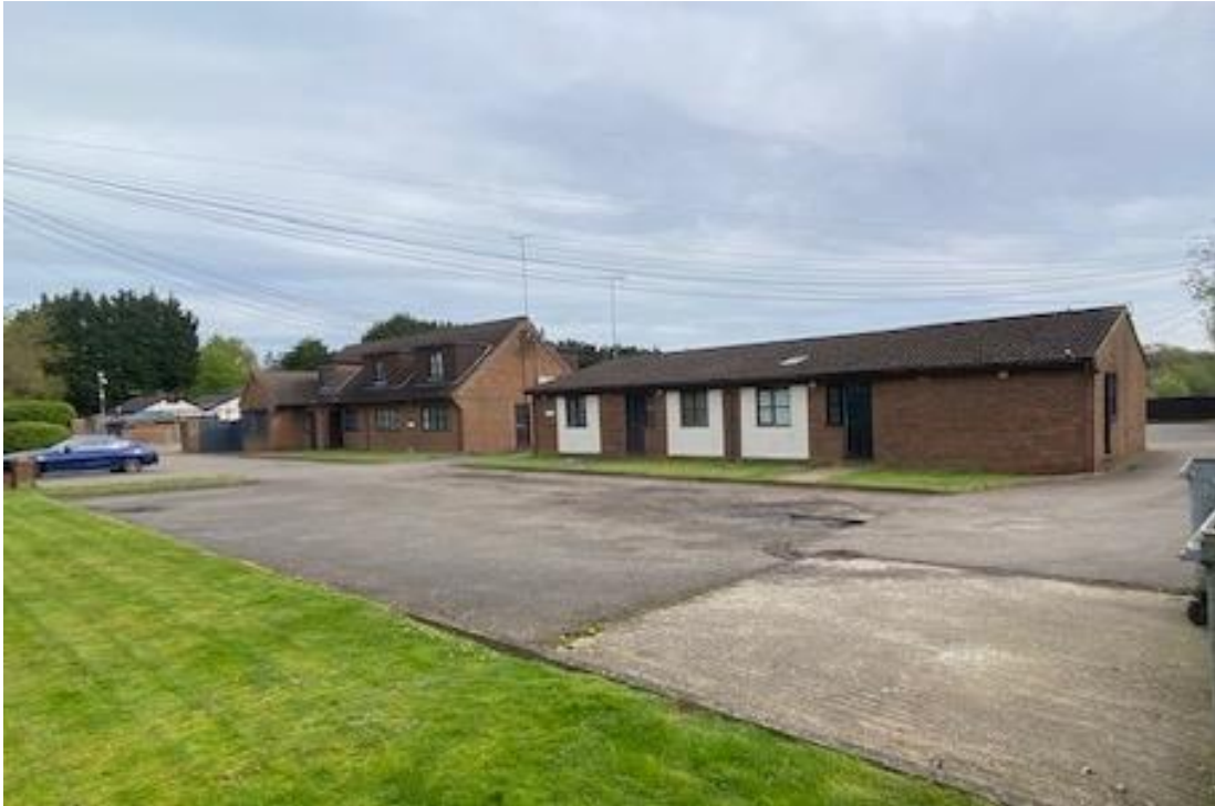
Building D and E (front looking east)
