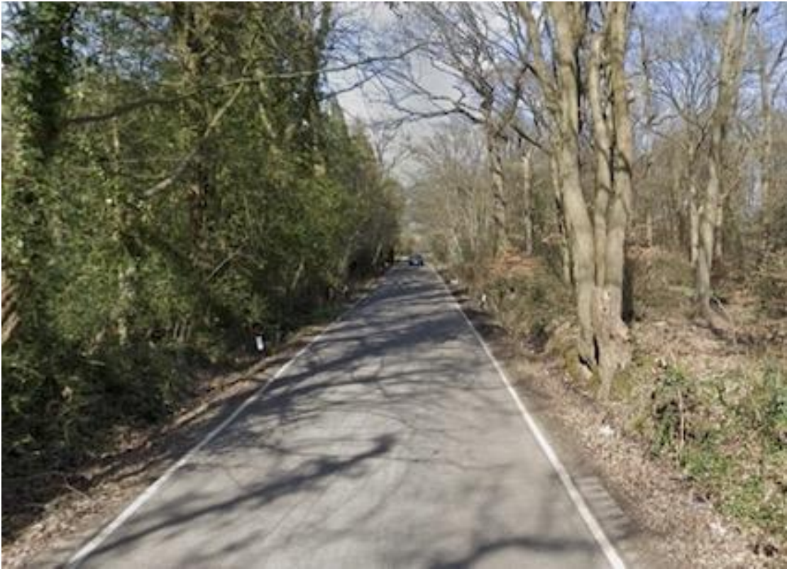
Lye Lane travelling north to M25 Bridge and Appeal Site
