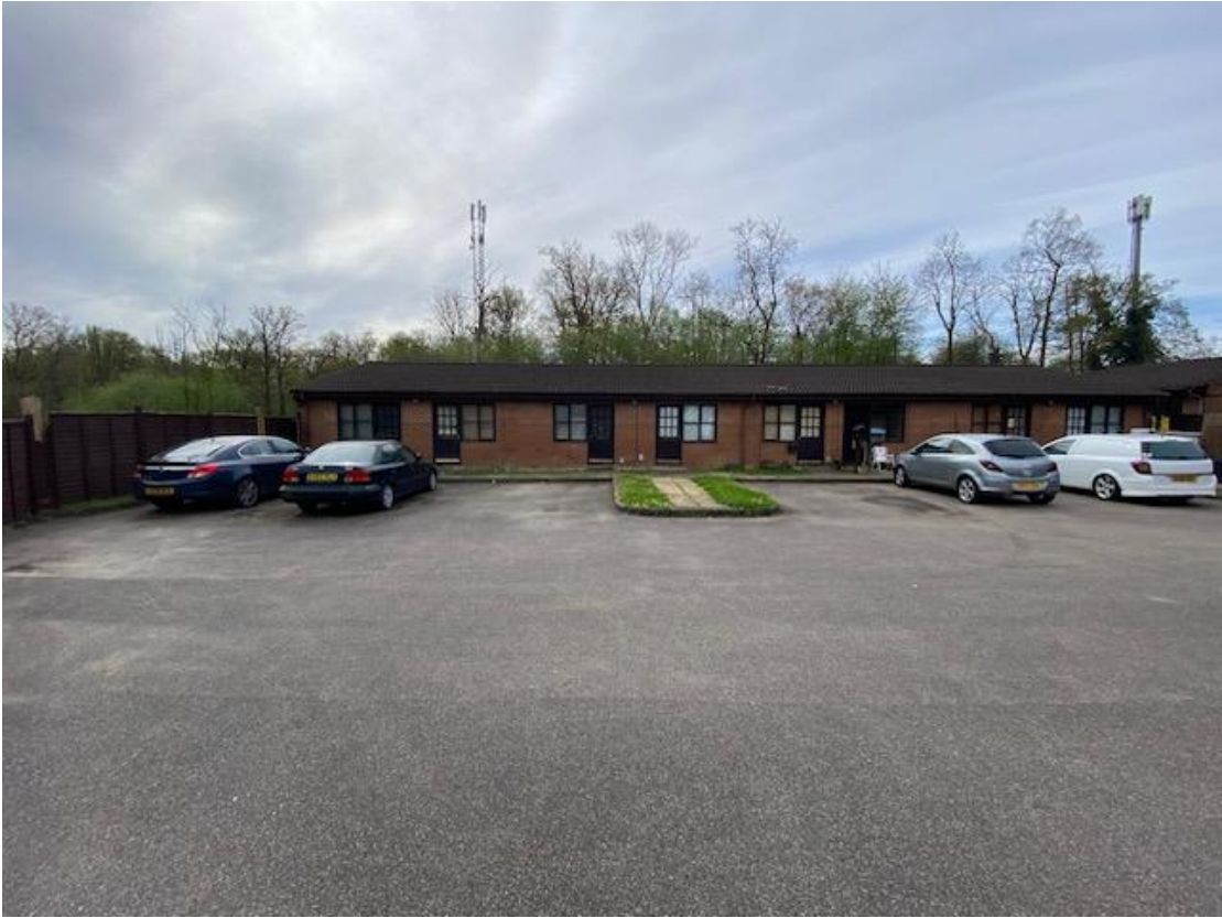
Building F looking south
