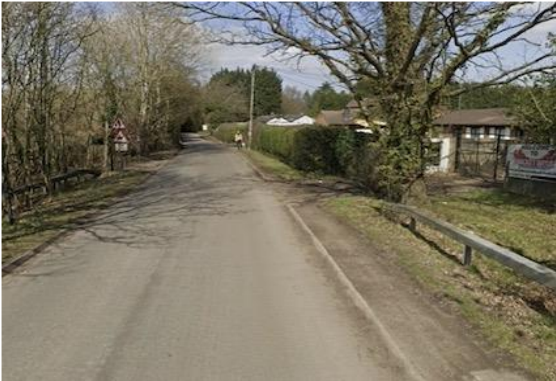
Site Frontage in location of the proposed acoustic fence looking north © Google
