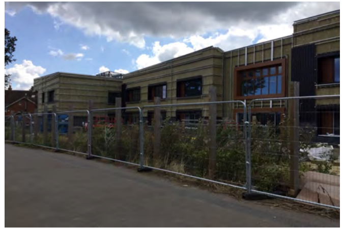
Looking west from south-east corner of sub-area with views of educational building under development
