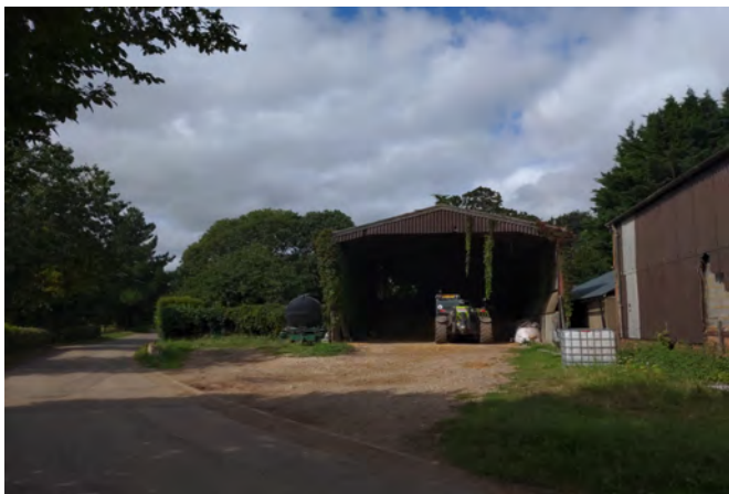
Looking east from Sandridgebury Lane at south boundary of the sub-area with views of agricultural buildings
