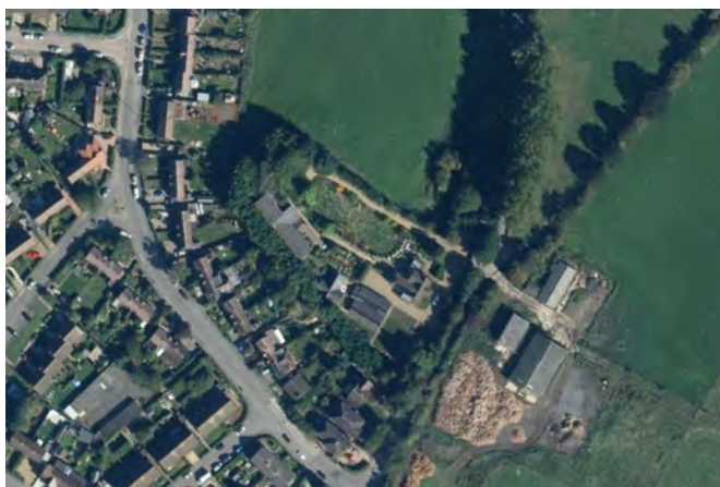
Aerial photography used as a result of limited access to and/or views of sub-area at the time of the site visit. (Bing Aerial, September 2021).
