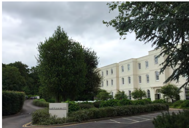
Looking south from north section of sub-area with views of hotel building
