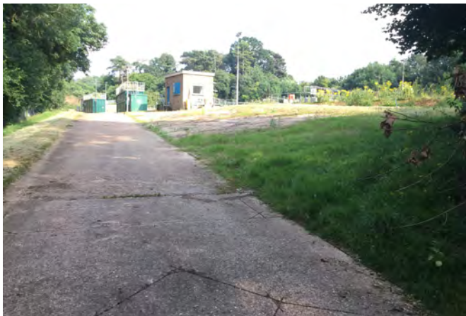
Looking east from the western boundary of the sub-area onto a water treatment plant.
