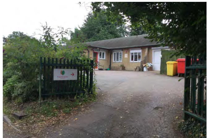
Looking south from the northern boundary onto a nursery
