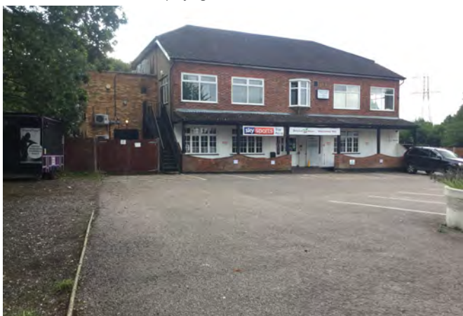
Looking east from the western boundary of the sub-area onto Bricket Wood Social Club and associated buildings and car park
