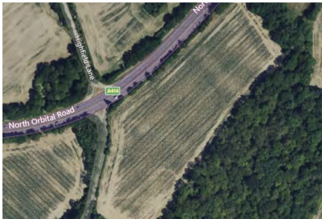
Aerial photography used as a result of limited access to and / or views of sub-area at the time of the site visit (Bing Aerial, September 2021)
