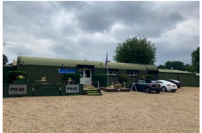
Looking south onto Radlett Golf Course club house in the north-east of the sub-area.
