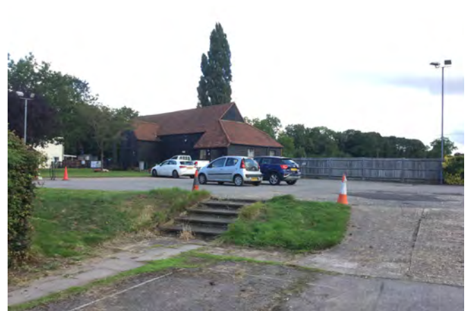
Looking north-west from the centre of the sub-area onto car park and parish church hall
