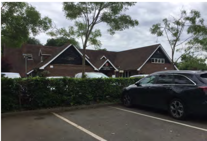
Looking onto Aldwickbury Park Golf Club clubhouse.
