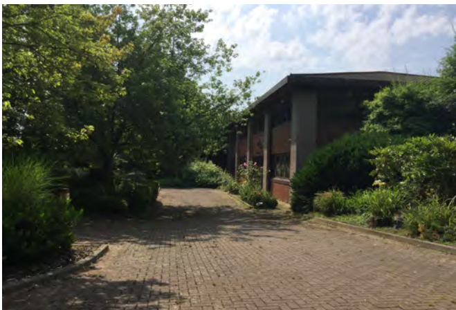
Looking south from the eastern boundary of the sub-area onto some commercial offices
