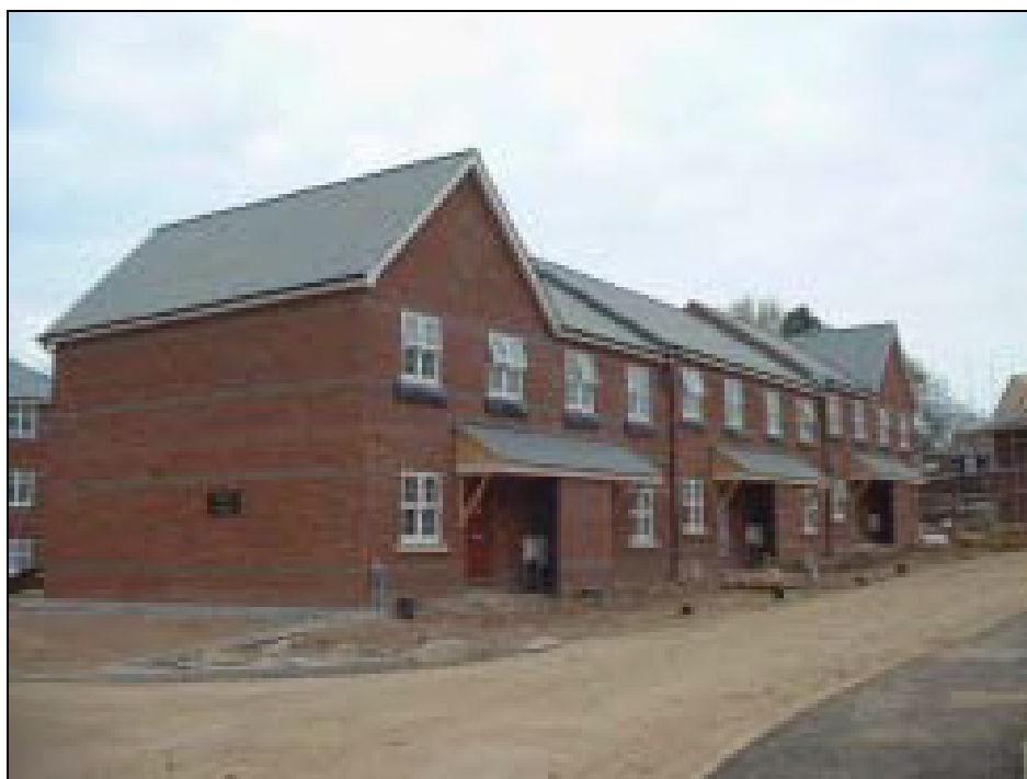
Affordable rented housing under construction, Napsbury Park, London Colney.
