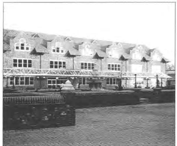
Victoria Square, St. Albans - New Offices
