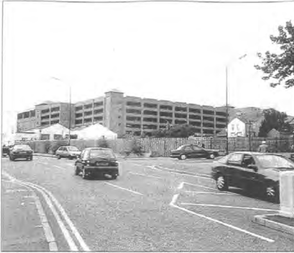
London Road/Marlborough Road - former Godfrey Davis Showroom site
