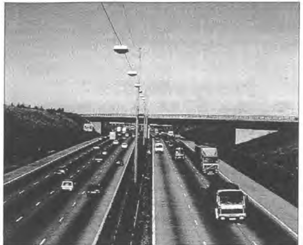
M1 Motorway at Junction 7
