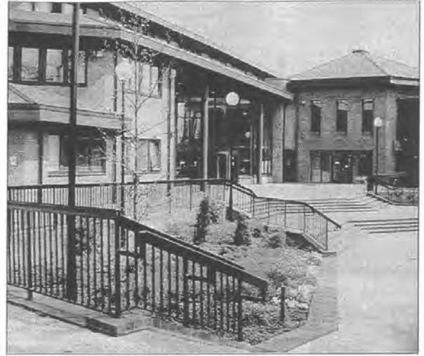
District Council Offices, Civic Centre
