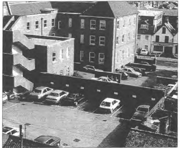
Rear of Victoria Street, St. Albans - business use parking
