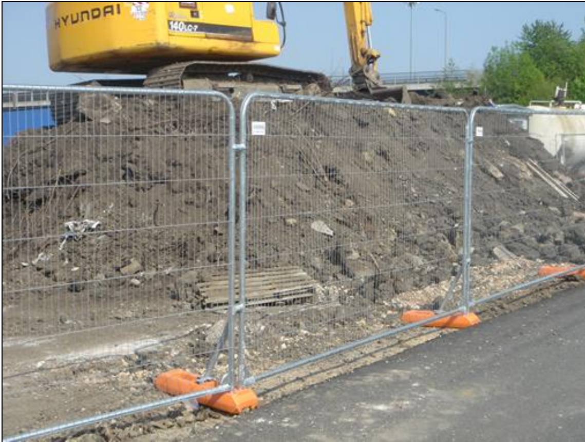
Photograph C – Example of Heras Tree Protective Fencing
