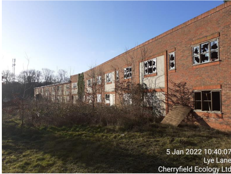
Figure 6: Rear elevation of B3
