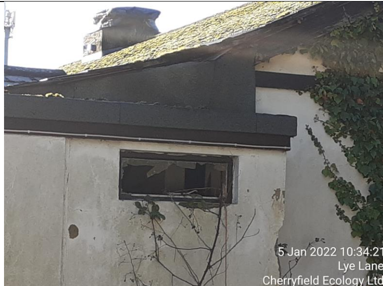
Figure 35: Example of access/exit point in window of B1
