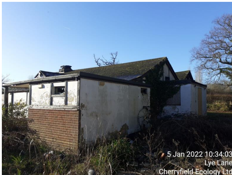
Figure 3: Rear elevation of B1
