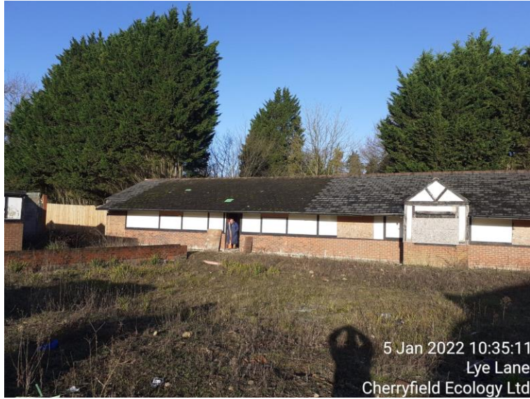
Figure 4: Front elevation of B2
