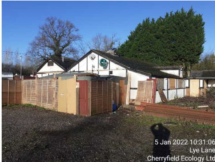
Figure 2: Front elevation of B1
