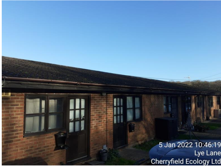
Figure 8: Front elevation of B5
