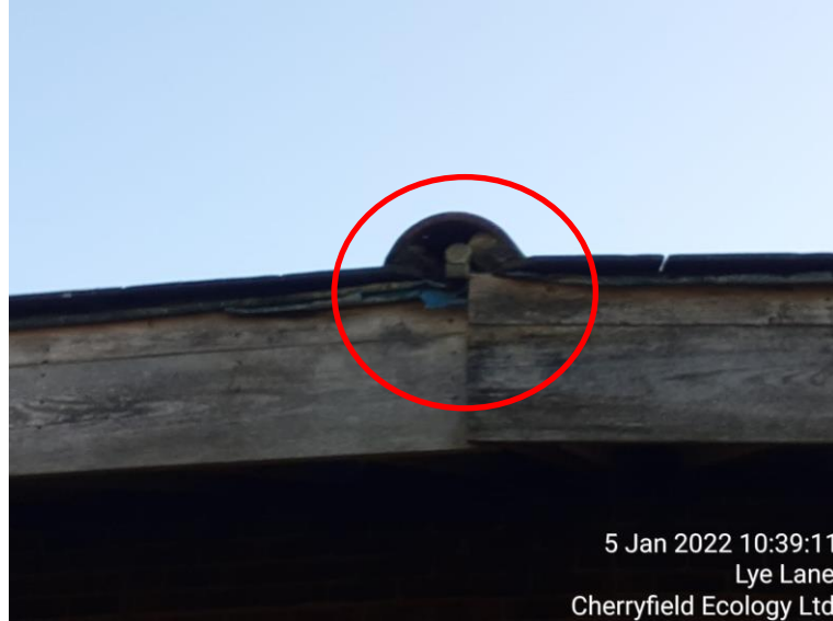
Figure 37: Example of gaps underneath the ridge tiles of B3
