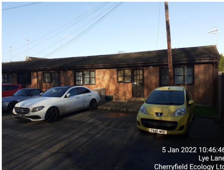
Figure 20: Example of hardstanding on site
