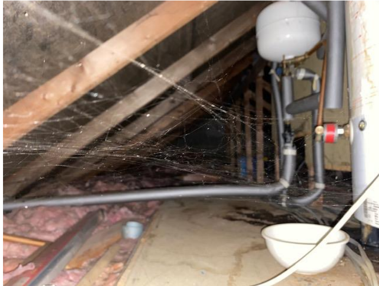
Figure 19: Example of a loft space within B8
