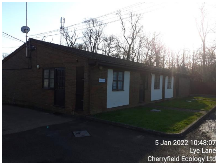
Figure 9: Front elevation of B6
