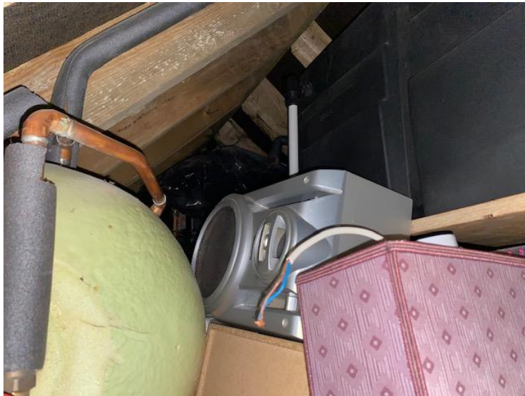
Figure 18: Example of a loft space within B7
