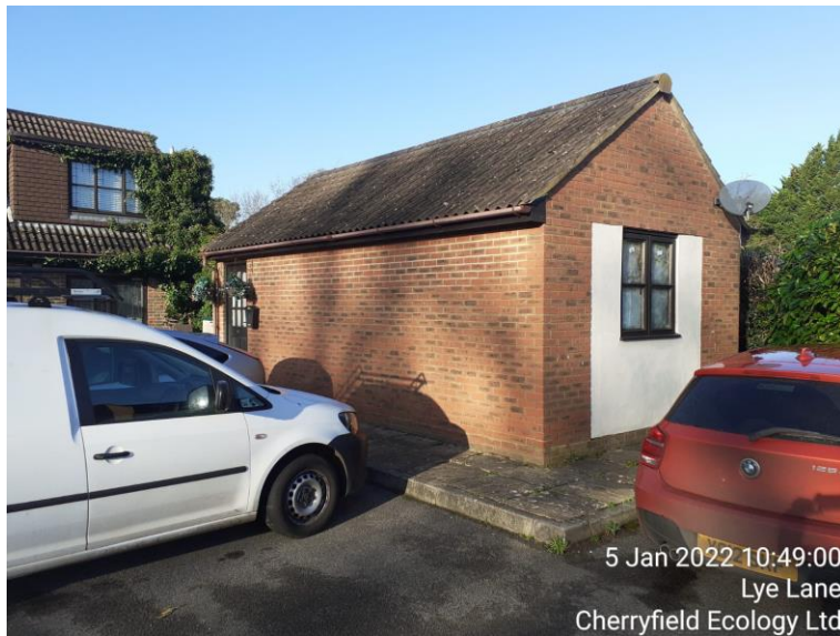
Figure 11: Front elevation of B8
