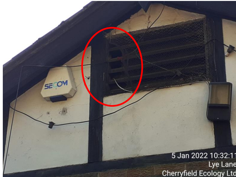
Figure 33: Example of access/exit point in air vent of B1
