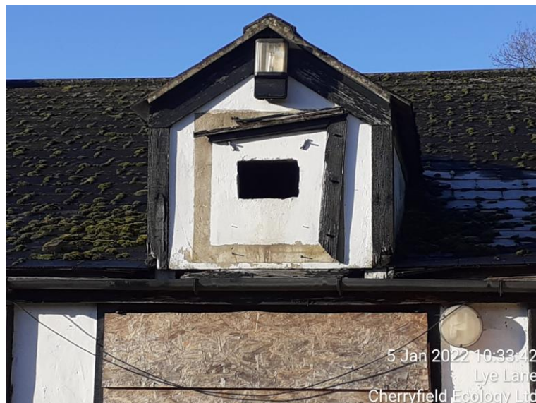
Figure 34: Example of access/exit point in dormer of B1
