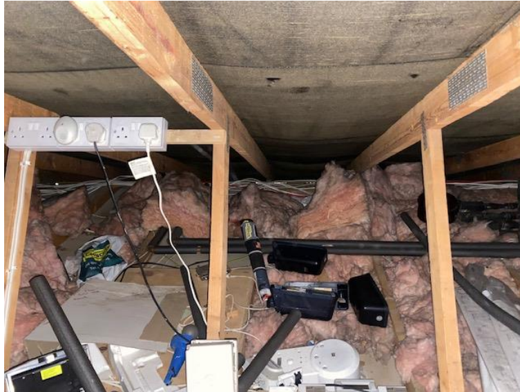
Figure 15: Loft space within B2
