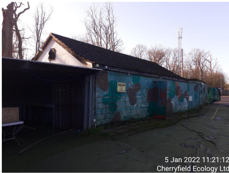
Figure 7: Front elevation of B4
