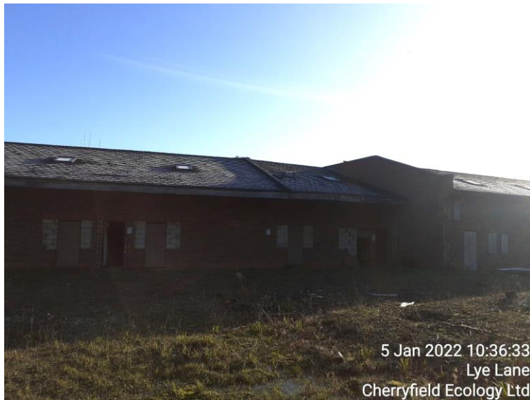
Figure 5: Front elevation of B3
