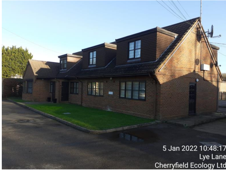
Figure 10: Front elevation of B7
