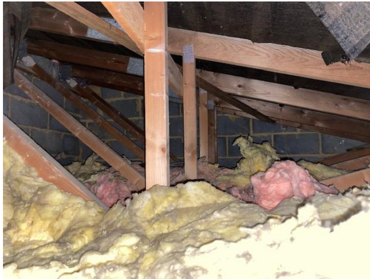
Figure 16: Example of a loft space within B5
