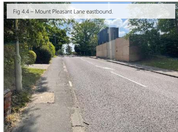
Wide carriageway, consider provision of an on-street cycle lane in line with LTN 1/20 guidance.
