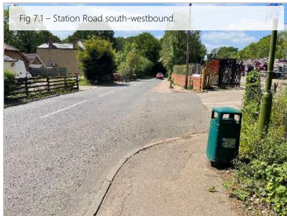
Consider provision of new uncontrolled pedestrian crossing comprising of dropped kerbs and tactile paving.
