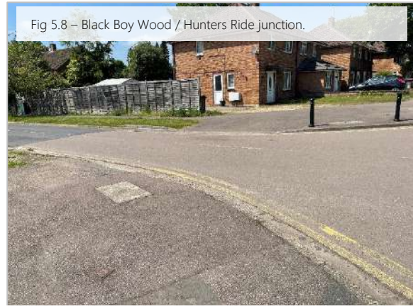
As per Fig 5.1, consider provision of new uncontrolled pedestrian crossing comprising of dropped kerbs and tactile paving.
