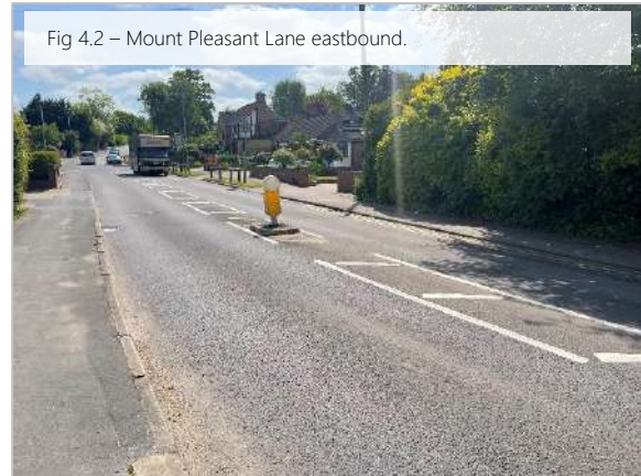
Consider provision of new uncontrolled crossing point with dropped kerbs, tactile paving, and refuge island.
