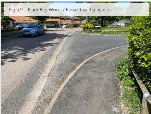
As per Fig 5.1, consider provision of new uncontrolled pedestrian crossing comprising of dropped kerbs and tactile paving.
