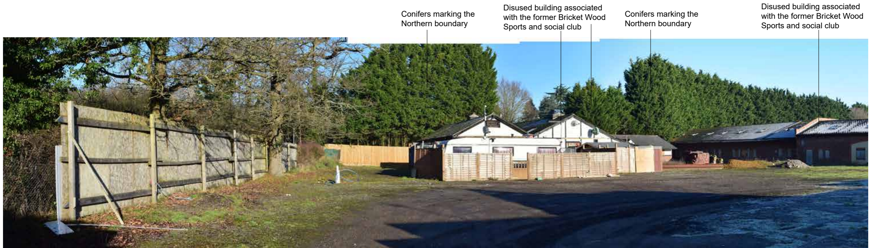
On-site View E - View from North West corner of the residential area of the site looking North across the site
