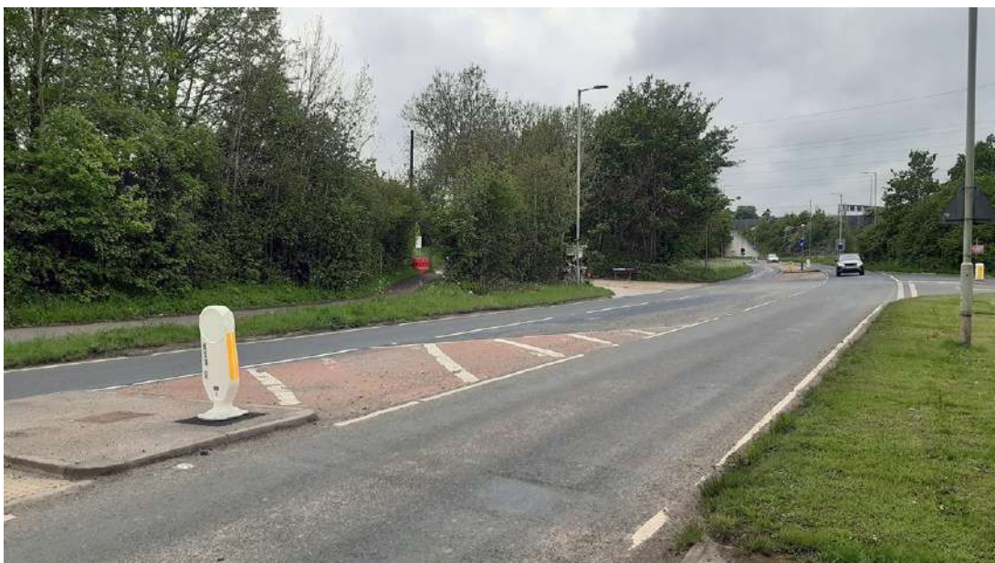
Figure 32: Existing crossing points on the Nickey Line to be improved – A5183 (top) and B487 (bottom)
