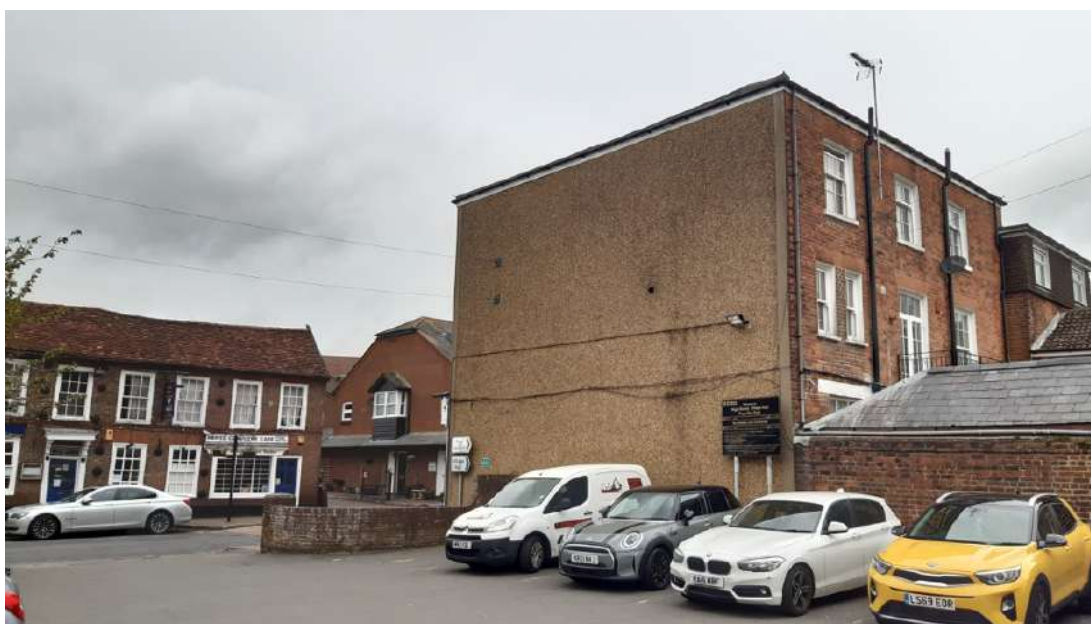
Figure 21: The Village Hall car park and blank end wall of buildings, which could be enlivened
