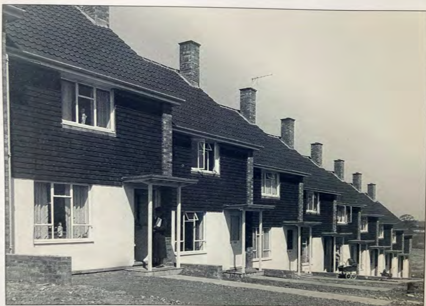
Newly completed houses at Galley Hill, Gadebridge.
