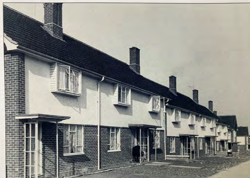
Houses in Warners End Road, newly completed in 1956.
