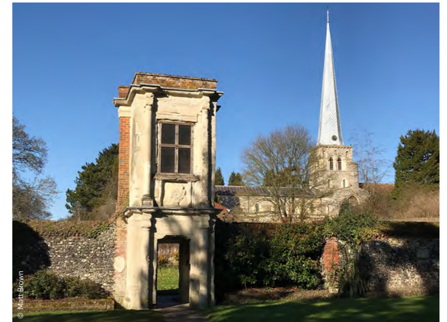
Historic structures - St Mary's Church and the Charter Tower
