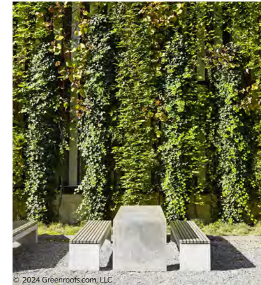
Trellis green wall
