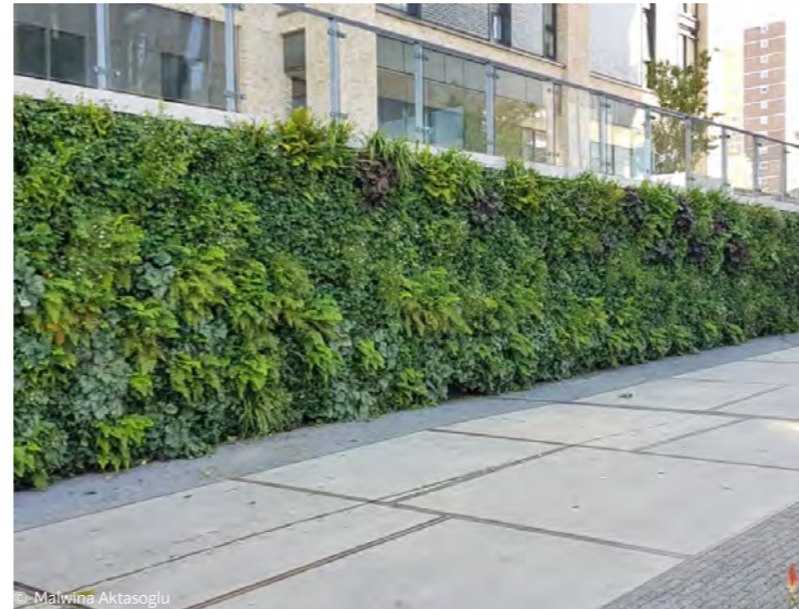
Living green wall within residential development platform
