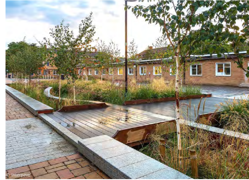
Rain gardens along residential streets
