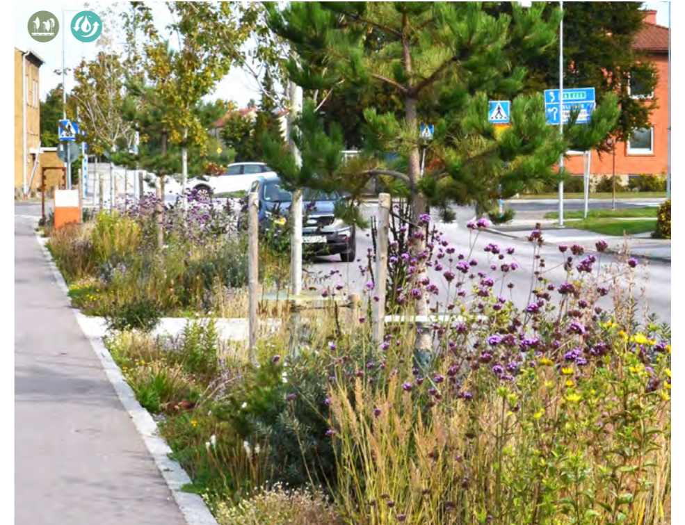
SuDS within residential streets/mews - rain gardens (Kingsbrook, Alysbury)
