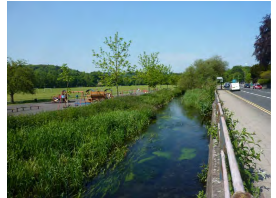
Deculverting waterways, Wye river, High Wycombe Town Centre
