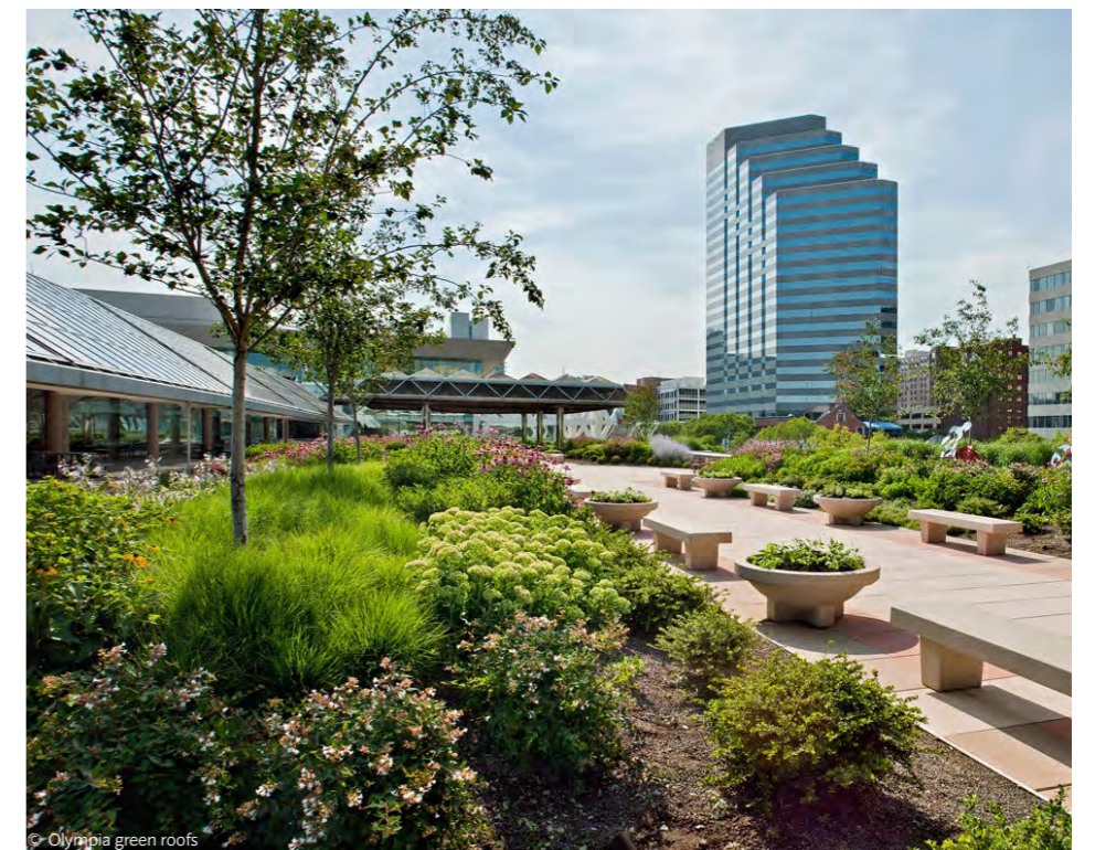
Intensive green roof - garden with variety of plants, seating spaces and accessible paths
