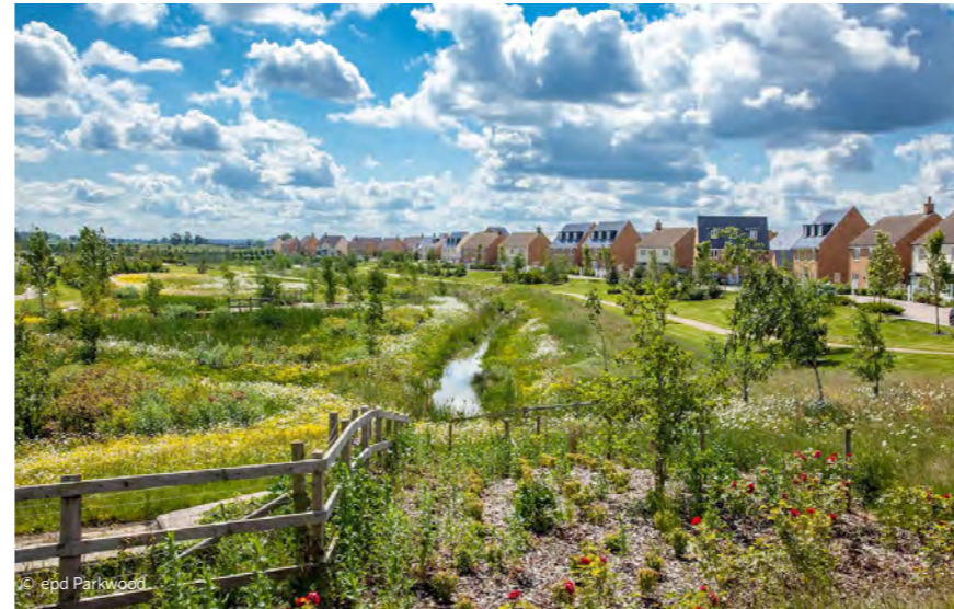
© epd Parkwood Sustainable drainage (Brooklands, Milton Keynes)
