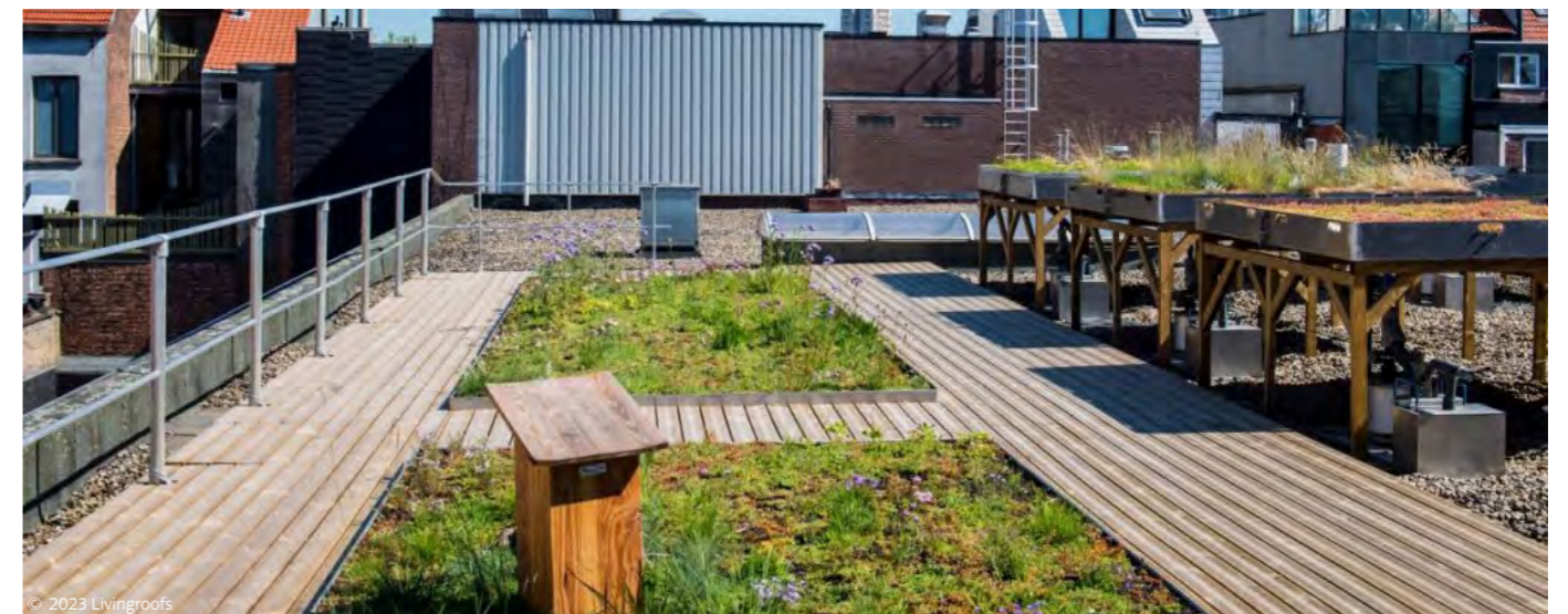
Blue green roof, Antwerp (Source- Livingroofs.org)
