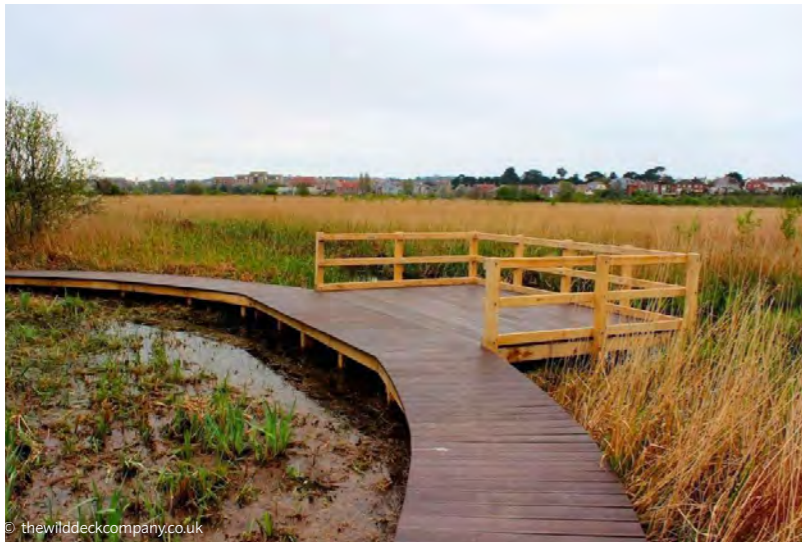
Accessible raised walkways with observation points/platforms
