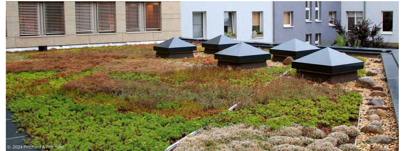
Extensive Blue roof (Source- Pritchard and Pritchard)
