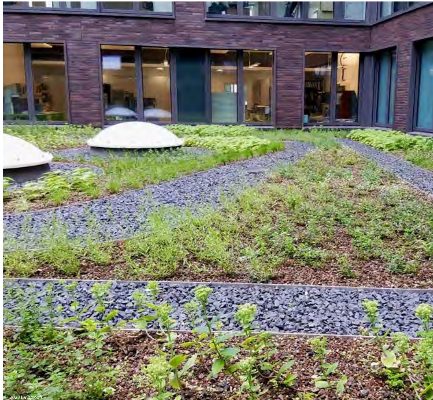
Intensive Blue Green Roof, Germany (Source- Livingroofs.org)
