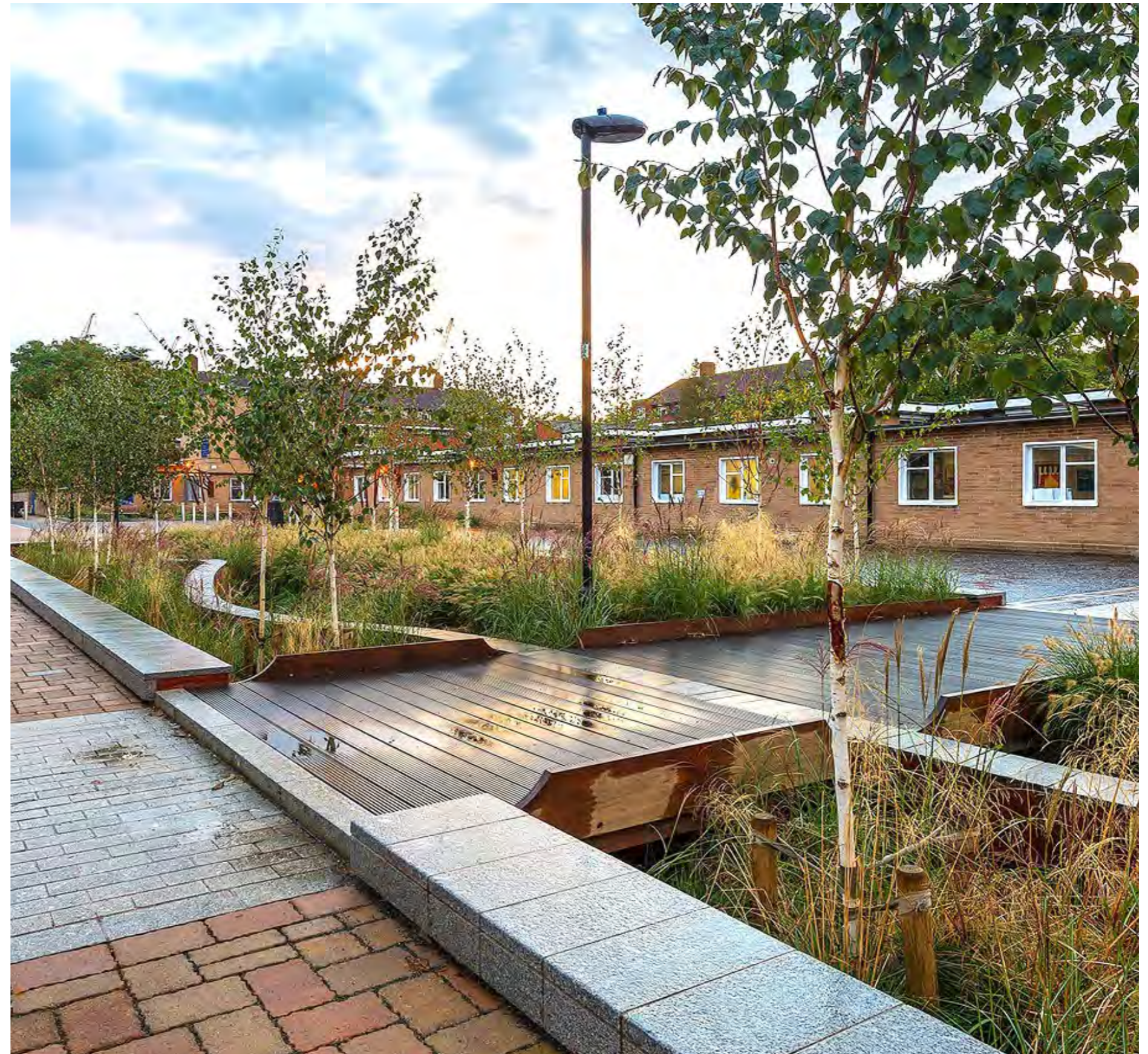
Nature-based Solution – a Sustainable Drainage System
