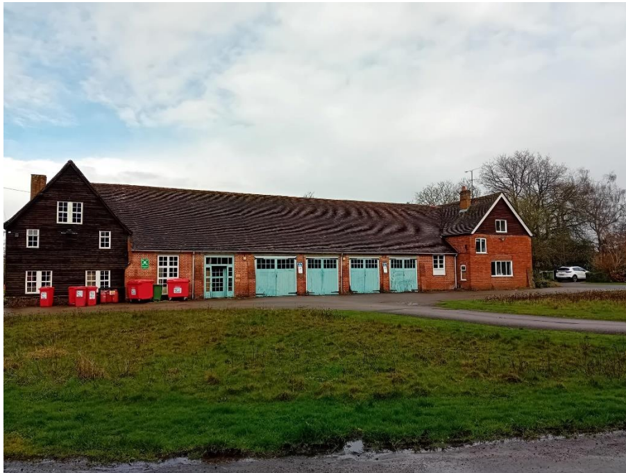
Figure 13 Storage barn to the east of Rothamsted Manor (left, with extensions)
