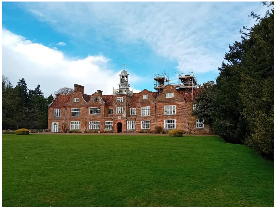
Figure 11 Front (west) elevation of Rothamsted Manor
