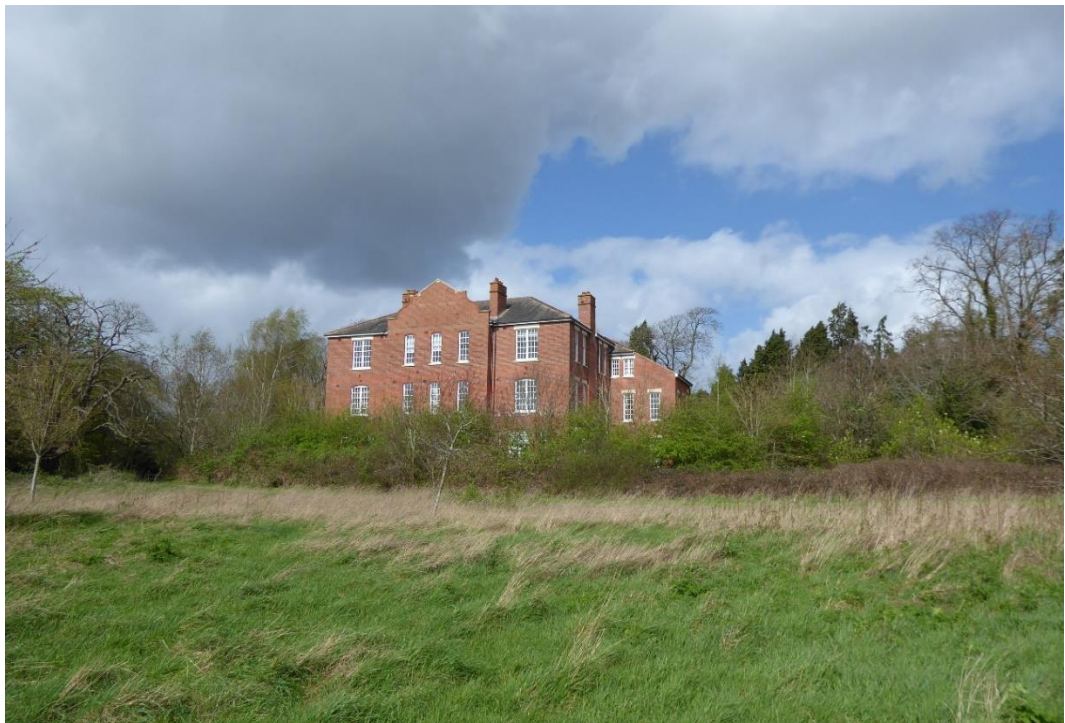
Figure 14 View north-west of one of the former detached villas within the southern portion of the park and garden
