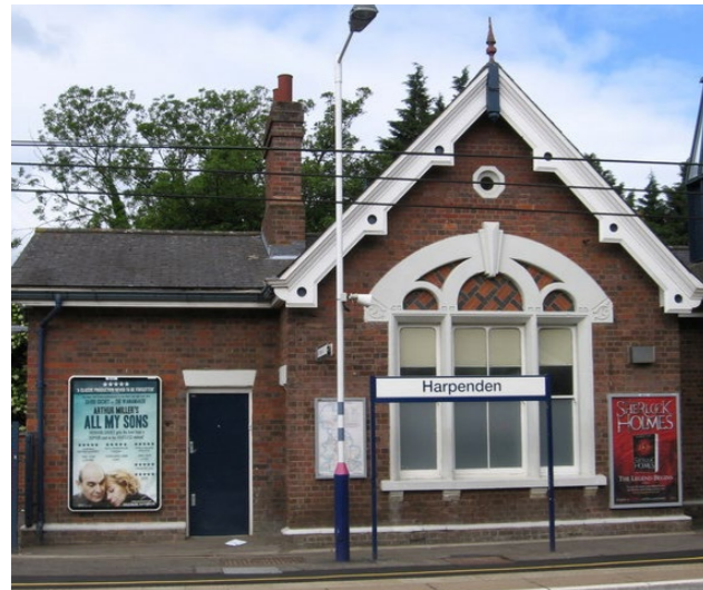
Fig 9: Harpenden Thameslink Rail Station
