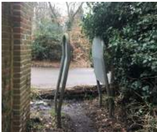
Figure 5 View of Footpath (St Stephen 018).
