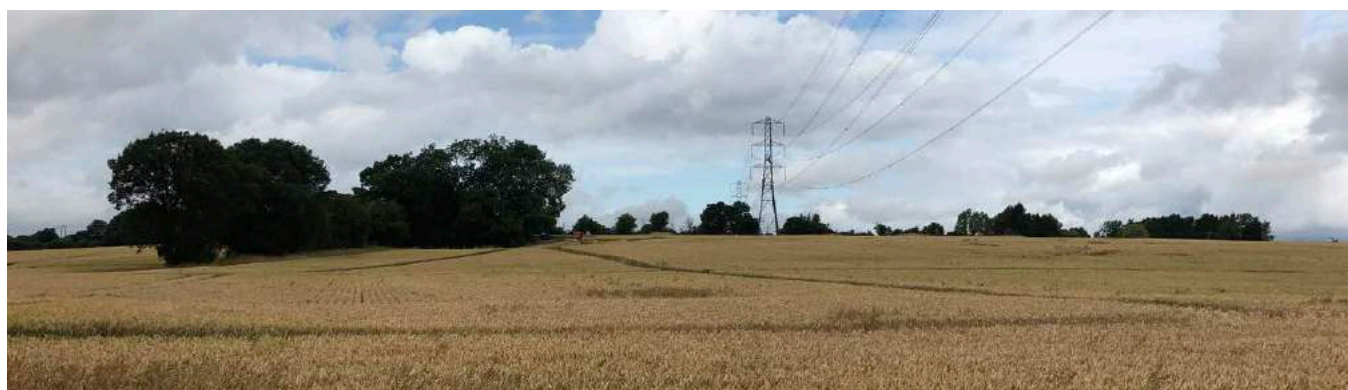
Pylons running along the western edge of the site and existing tree belts
