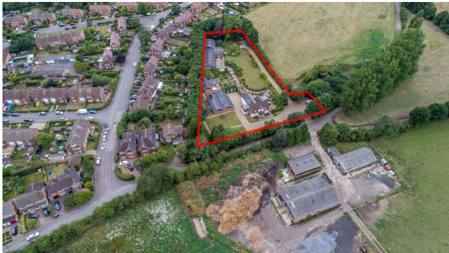
Figure 1: Sauncey View Lodge site looking north-west
