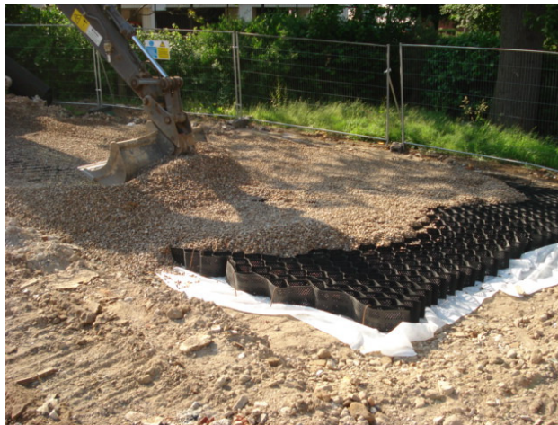
Figure 1. Installed 3D Webbing system around retained existing trees.
