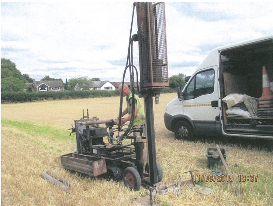
Photo 16: view of WS9 during drilling, looking north-east.
