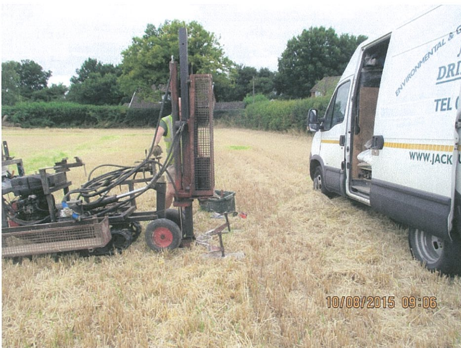
Photo 6: view of WS2 during drilling, looking north.
