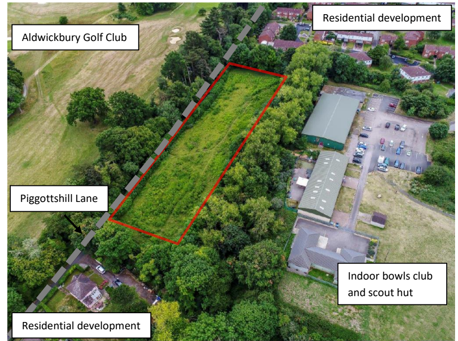
Figure 2: Aerial Imagery of the Site
