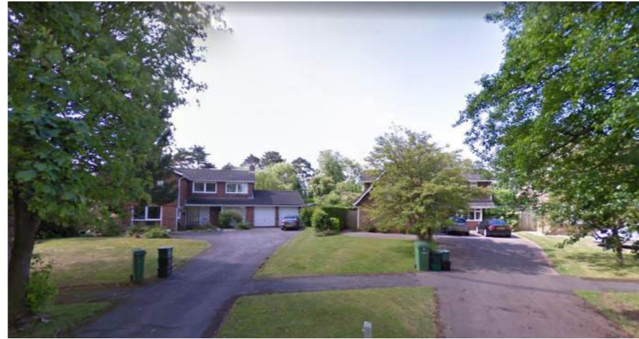
View 4 - Two storey houses along The Deerings
