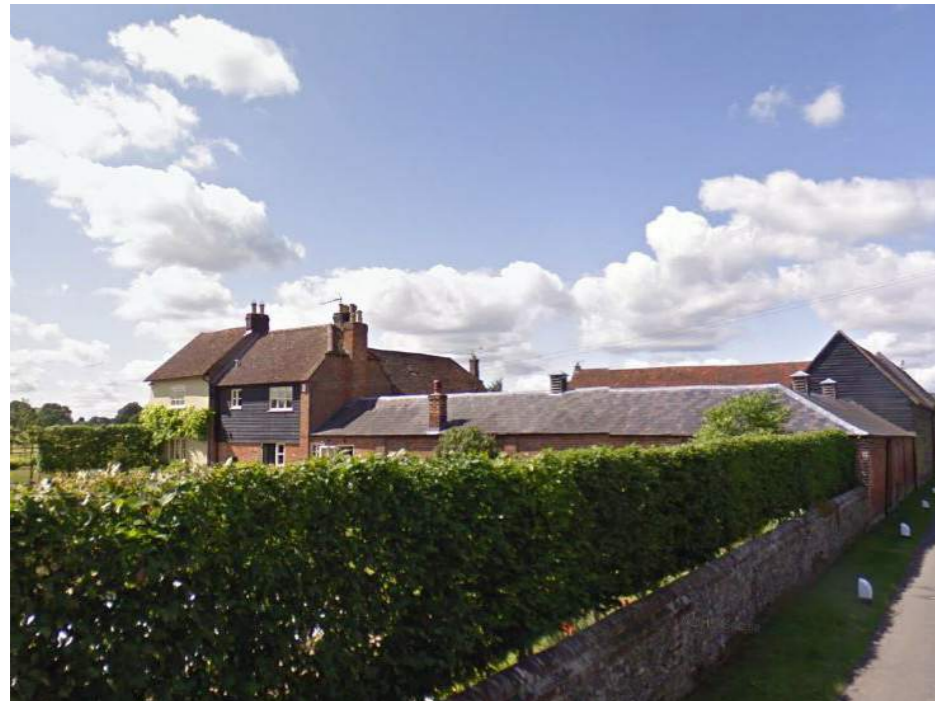
Listed Building A - Beeson House
