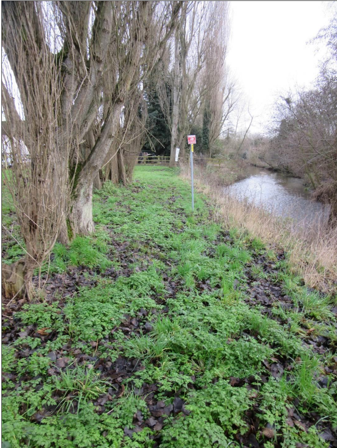
Photograph C – Showing Poplars adjacent to River Lee which will restrict the root activity of these trees
