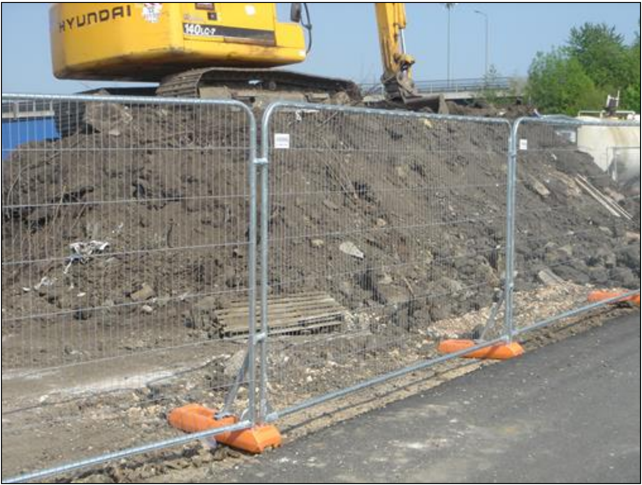
Photograph D – Example of Heras Tree Protective Fencing
