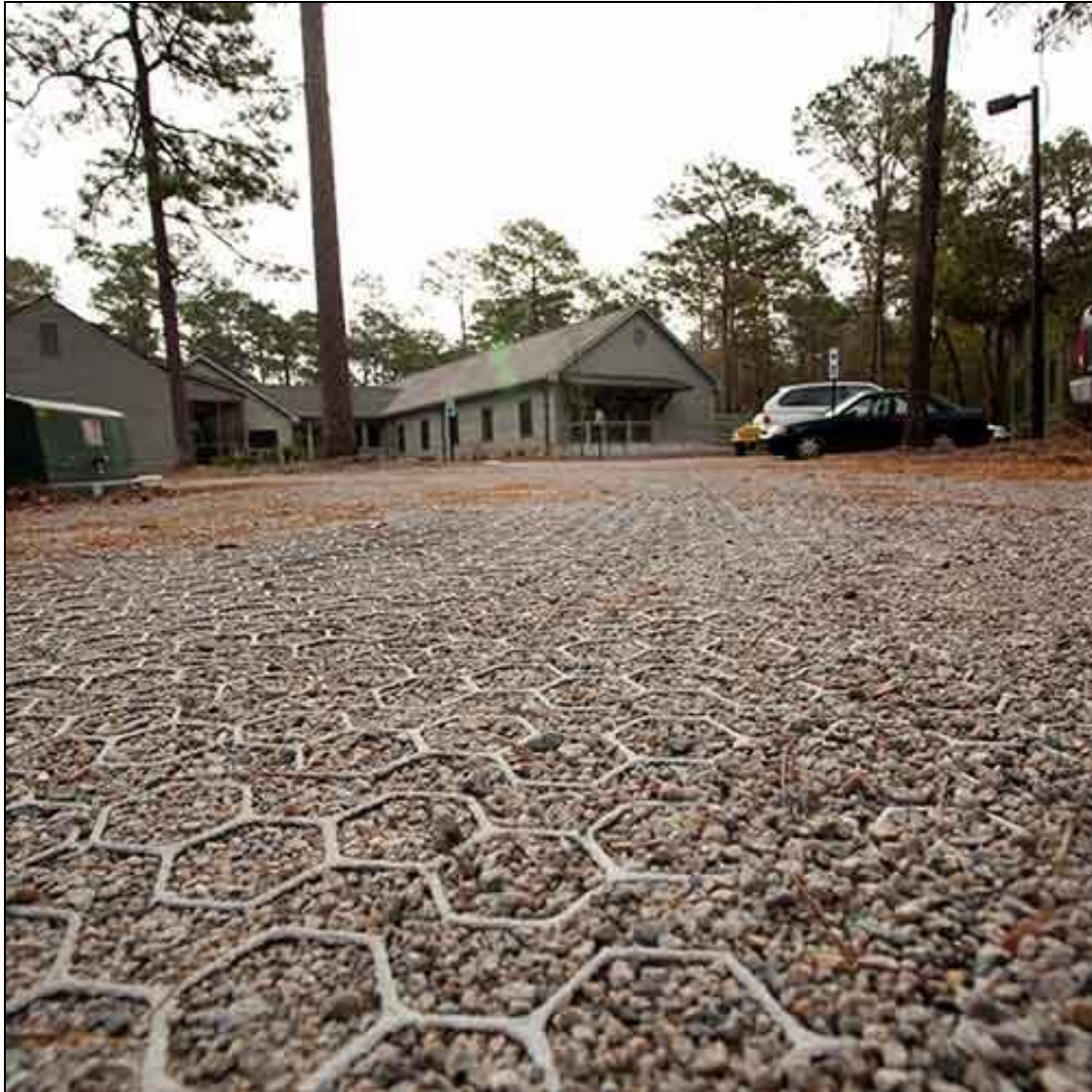
Photograph E – Geo Cell with gravel infill.
