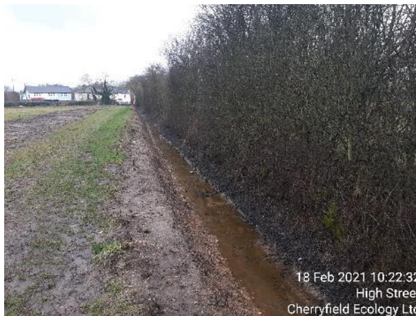
Figure 16: Newly created ditch within site boundary.
