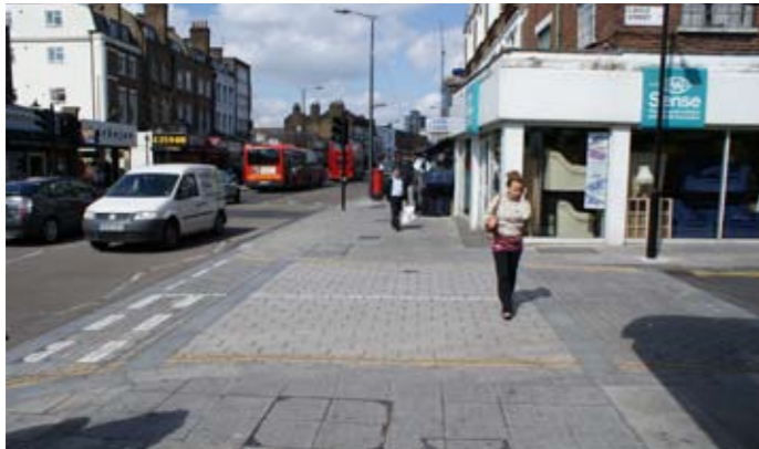
Side road entry treatments offer pedestrians additional priority and comfort
