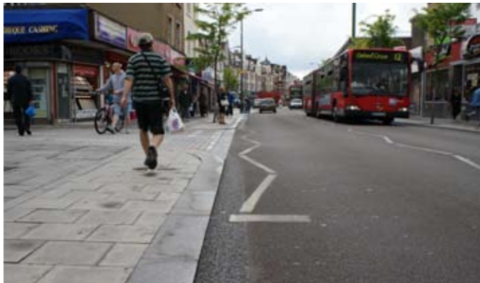
Low kerb heights can improve pedestrian crossing and help to change the character of a street
