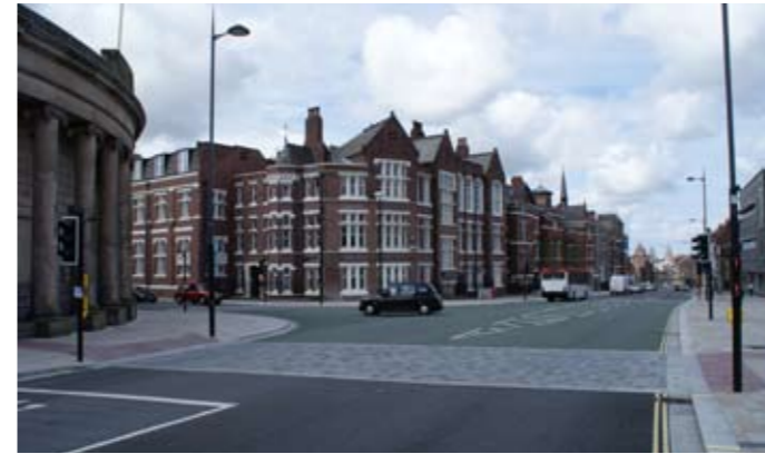
Use of contrasting materials can help to raise the profile of a junction
