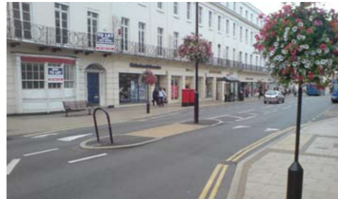
Informal crossing points can be a useful addition where formal facilities are not appropriate
