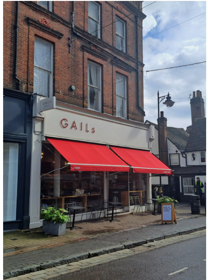
The awnings on this shopfront are detailed to fold neatly into the fascia, so whether closed or open the shopfront is not obscured.
