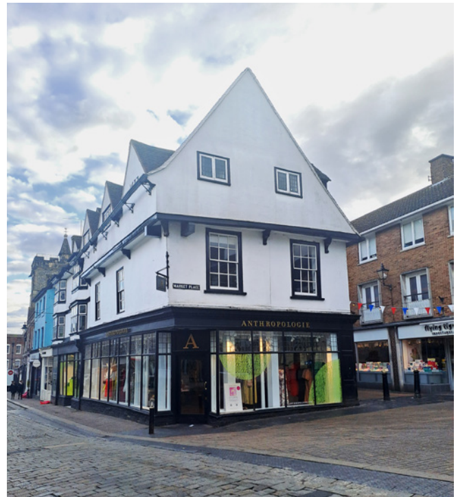
The corporate branding on this shop has been tailored to better suit the existing building.
