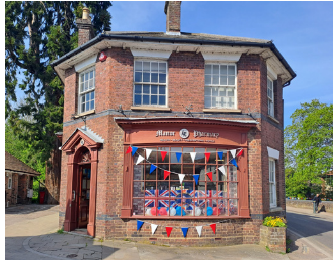
This shopfront window is broken up with glazing panes in the same proportions as the upper floor sash windows.
