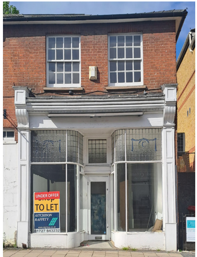
This shopfront helps visually support the building above, balancing out the elongated proportions of its early shopfront. The panelling details on the pilasters correspond to the glazing details and fascia creating a coherent design.
