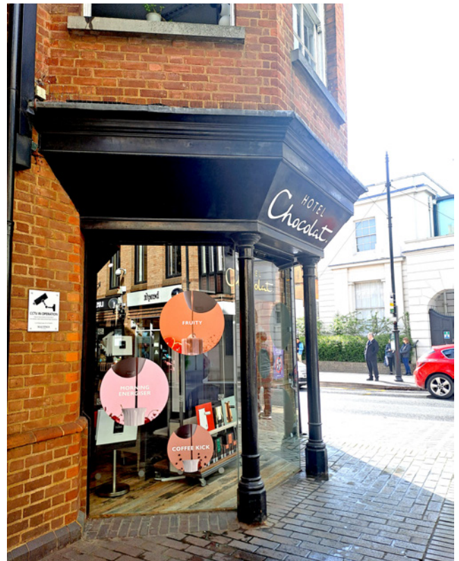
This modern shopfront does not have a stallriser, but the columns and fascia details help give visual support to the upper floors.
