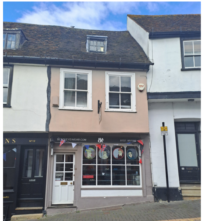
The alarm box on this building has been placed at high level on the window away from the hanging sign and small scale fascia.
