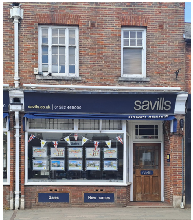
The stallriser on this shop is formed of brick and thin terracotta tiles which match the detailing on the rest of the building.
