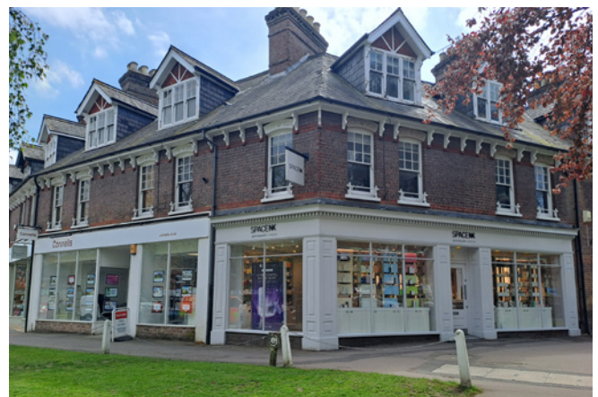
The cornice on the corner shopfront creates a better relationship with the upper floors of this building than its neighbour.
