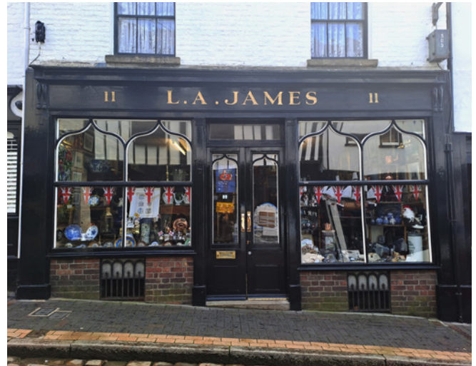
No. 11 George Street retains its highly attractive Victorian shopfront with decorative ogee arches. The fascia is in proportion with the rest of the shopfront and building.
