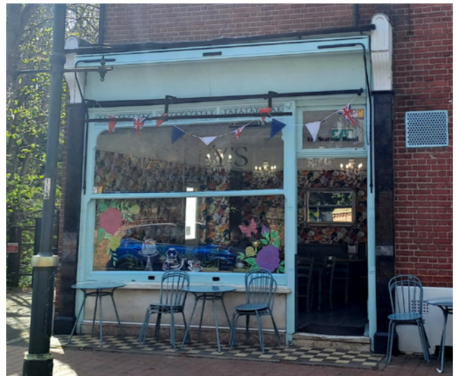
This shopfront window has a traditional decorative grille associated with C19 greengrocer and produce shops and a mullion to break up the large extent of glazing.
