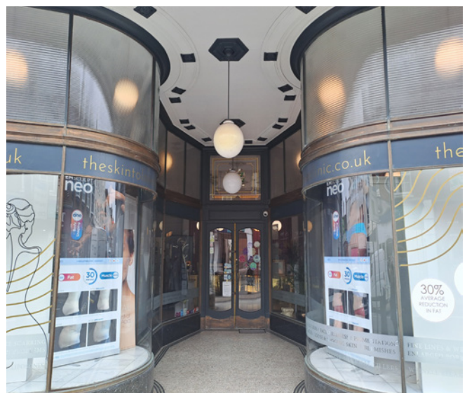
This decorative recessed doorway has a panelled soffit and decorative tile floor.
