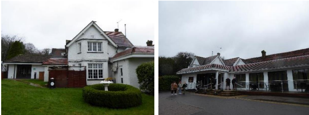
Figure 14 Aubrey Park Hotel and extensions to the hotel with historic roof structure and chimney visible above modern extension
