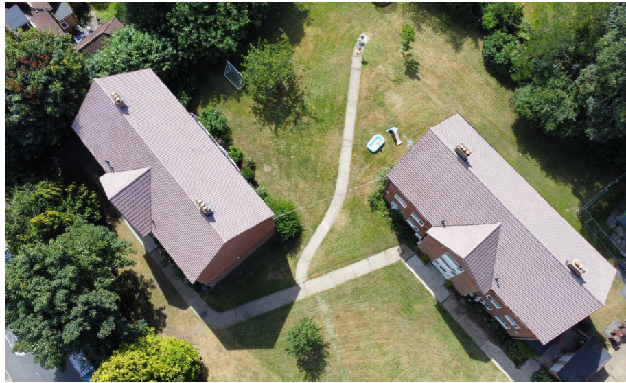
Completed Roof Renewals – Hall Place Close, St Albans (Aerial view)
