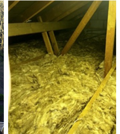
Upgraded loft insulation
