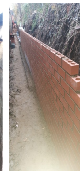
Ladies Grove Garages, St Albans – Retaining wall installed to rear of garage blocks
