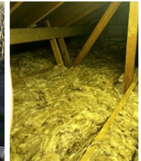
Upgraded loft insulation
