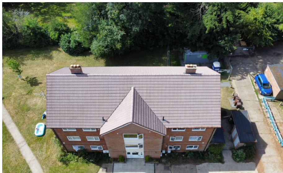
Completed Roof Renewals – Hall Place Close, St Albans
