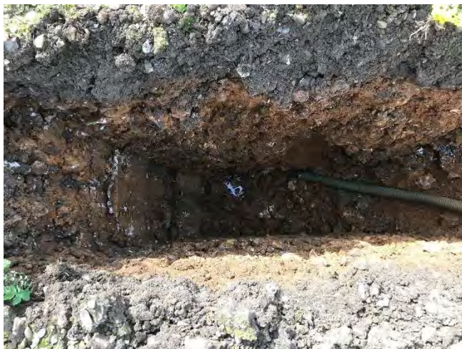
Photo 3: Excavation of trial pit IT02.
