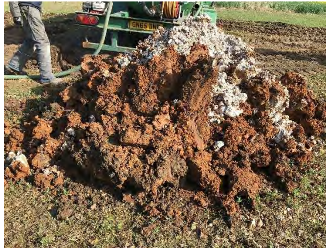
Photo 2: Arisings from trial pit IT01.
