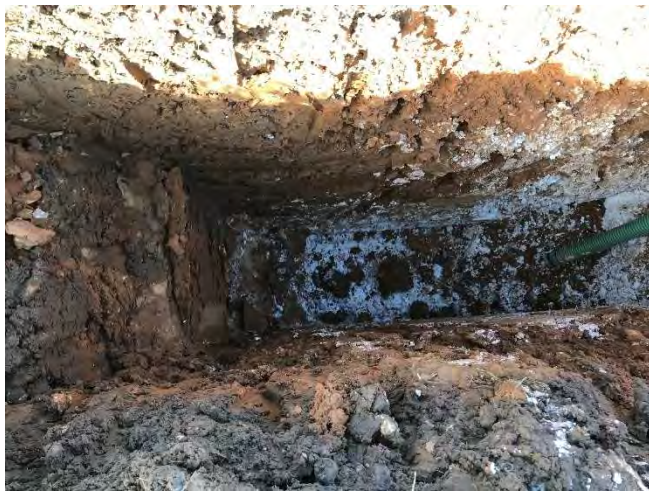
Photo 1: Excavation of trial pit IT01.
