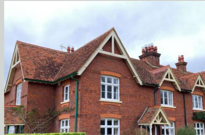
Gable forms with timber detailing
