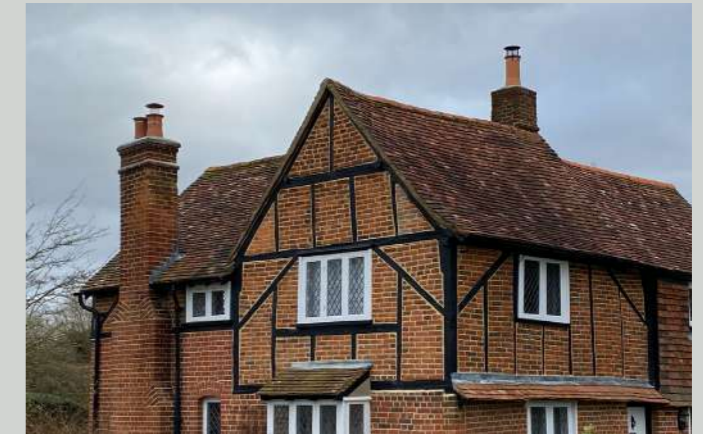
Tall chimney stacks
