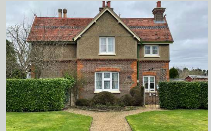
Brickwork detailing on corners and use of brick banding at storey heights
