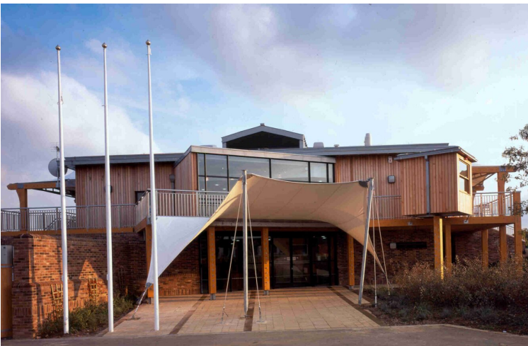
Existing Old Albanians Sports Association (OASA) Pavilion. Original Planning approval for 2,300m 2 facility, later reduced 1,600m 2 . Note materials including vertical timber cladding, masonry, aluminium framed glazing, raised seam roof with rooflights.
