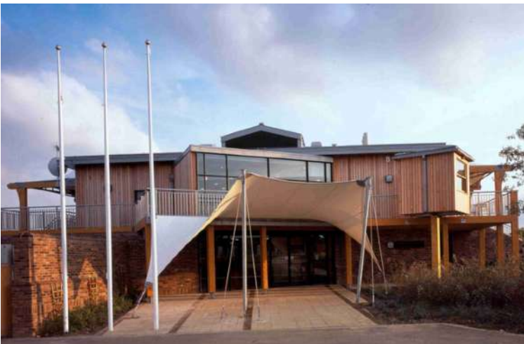
Existing Old Albanians Sports Association (OASA) Pavilion. Original Planning approval for 2,300m 2 facility, later reduced 1,600m 2 . Note materials including vertical timber cladding, masonry, aluminium framed glazing, raised seam roof with rooflights.
