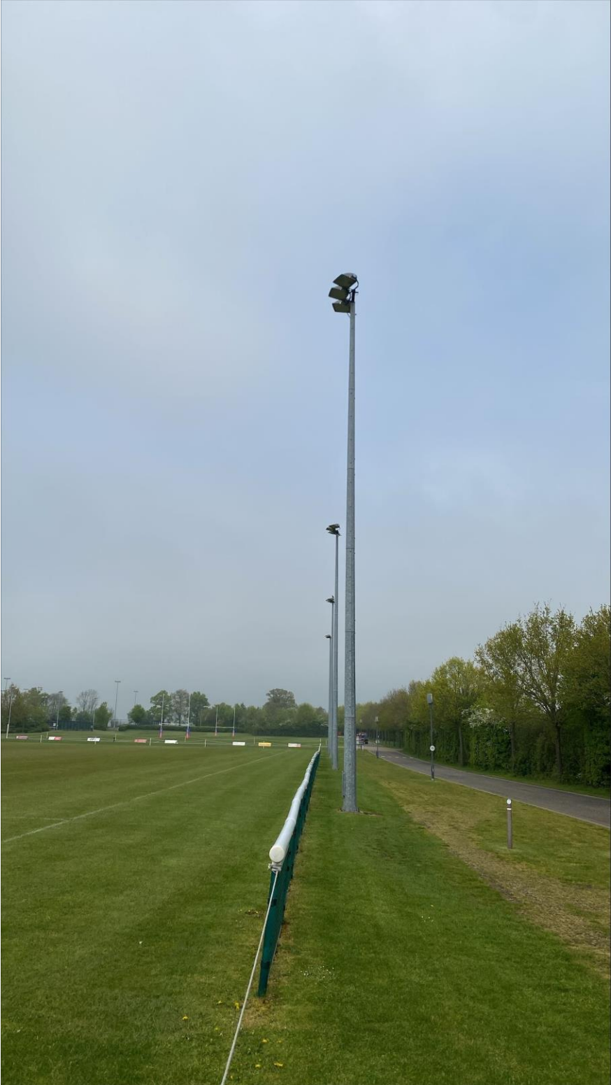
Three head floodlights on 16m column on match pitch
