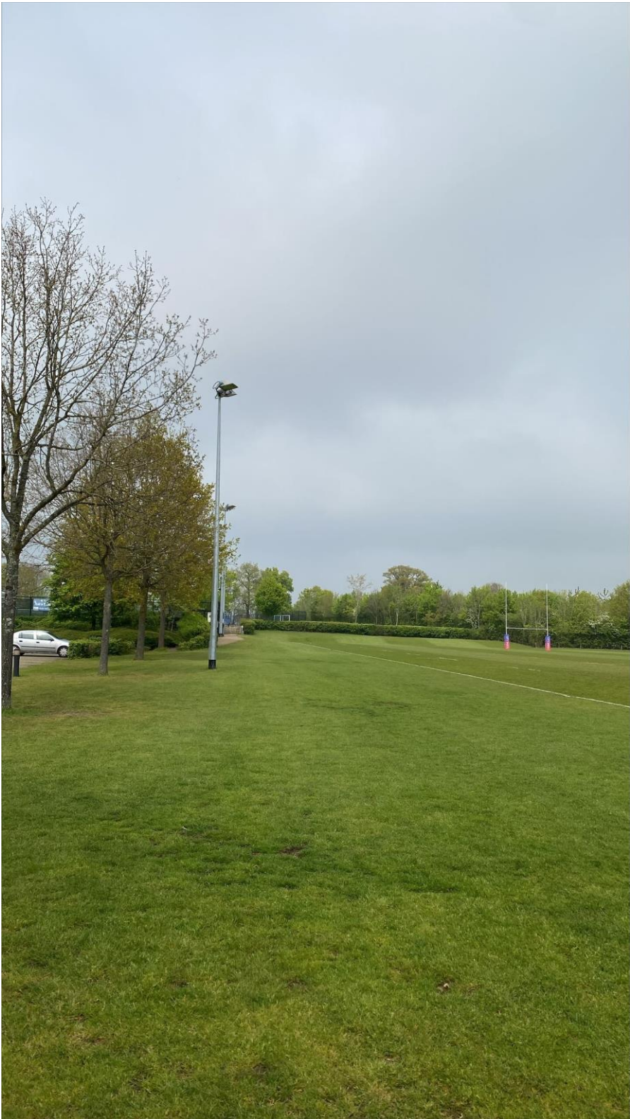
Twin Head floodlights on 16m column on training pitch
