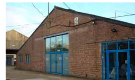
(H) Engineering Workshop
