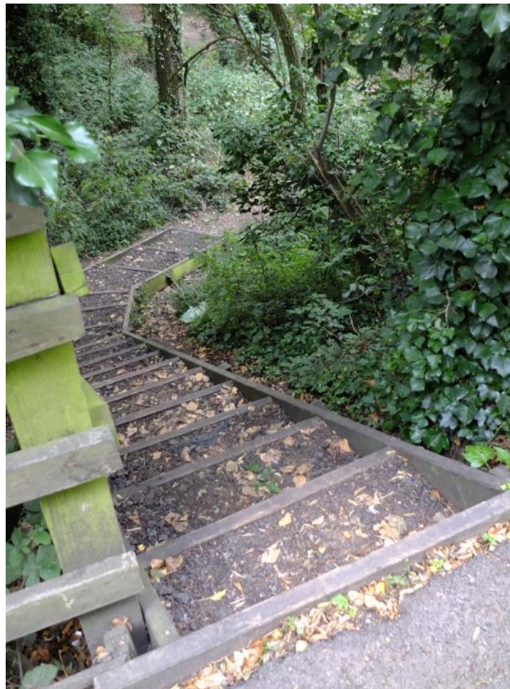
△ Access steps to the Nickey Line from Cherry Tree Lane
